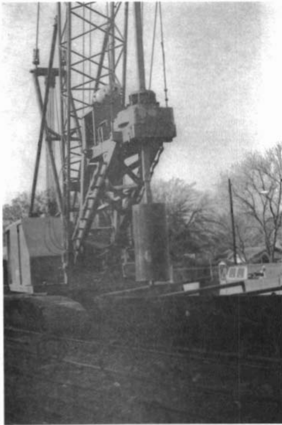
Fig. 5.11. Extracting bentonite slurry from within steel casing using plunger-type bucket.
