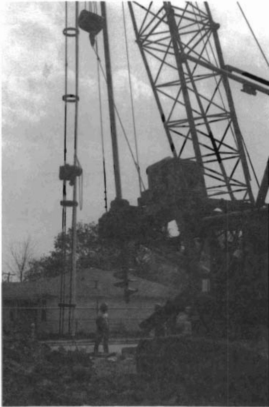
Fig. 5.17. Installing instrumented reinforcing cage with attached soil inclusion "defect".
