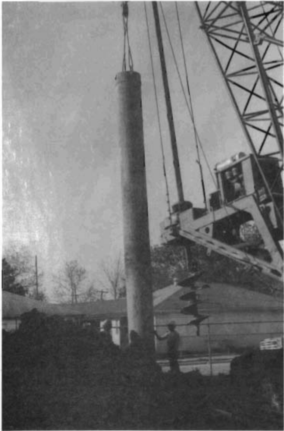
Fig. 5.10. Installing 30-in. (76.2 cm) diameter steel casing in augered hole.
