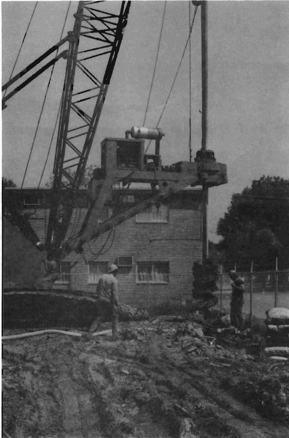
Fig 5.8. Drilling 50 ft. (15.2 m) pier shaft using 32 in. (81.3 cm) diameter auger.
