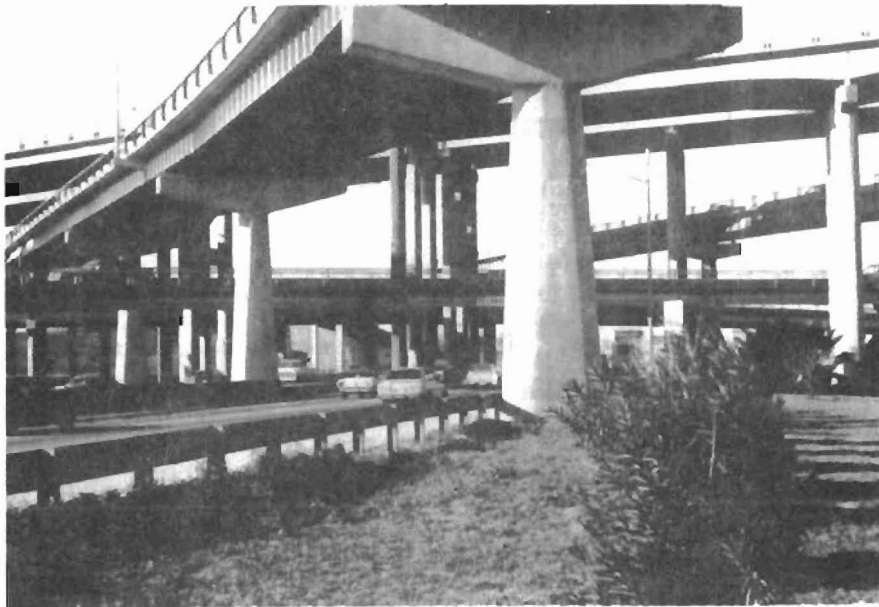
(a) In a busy highway exchange
