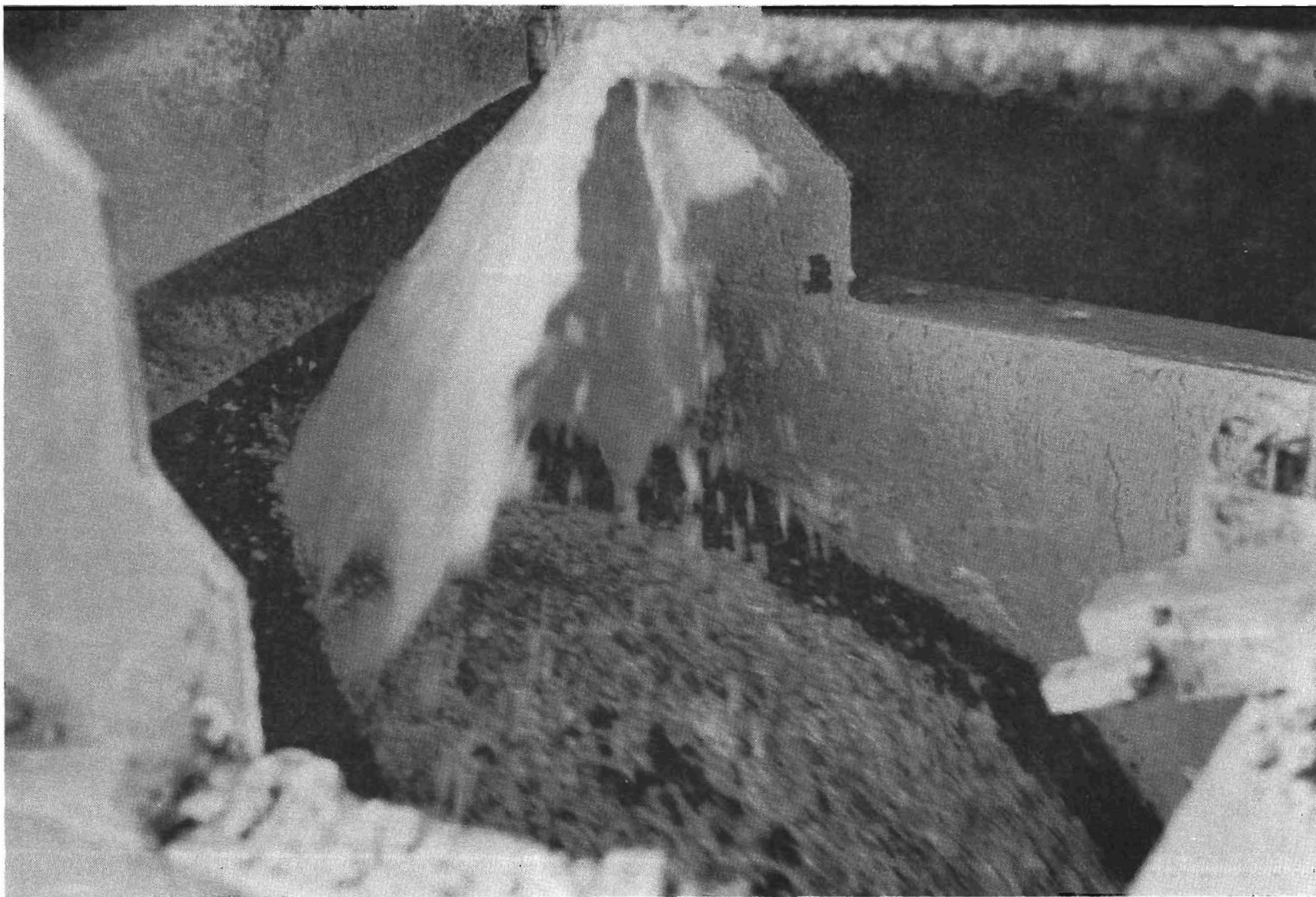
Fig 33. Lime slurry being applied to the cold feed (Texas plant).
