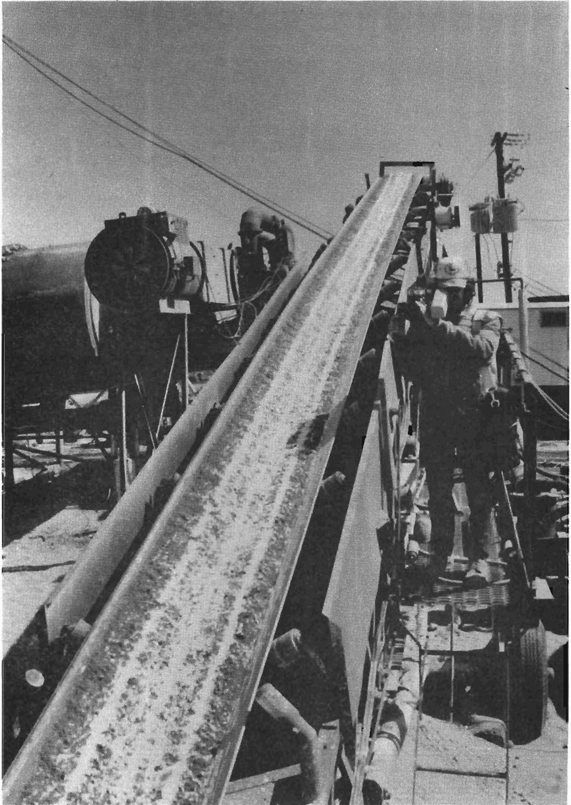
Fig 34. Application of lime slurry to aggregate on the cold feed belt.
