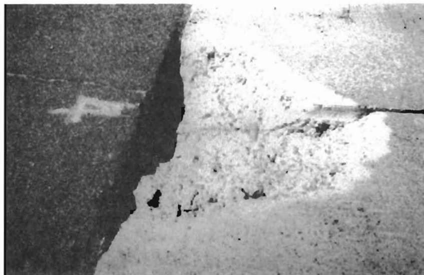
Fig. 4.2 Repair Area After Sandblasting.
