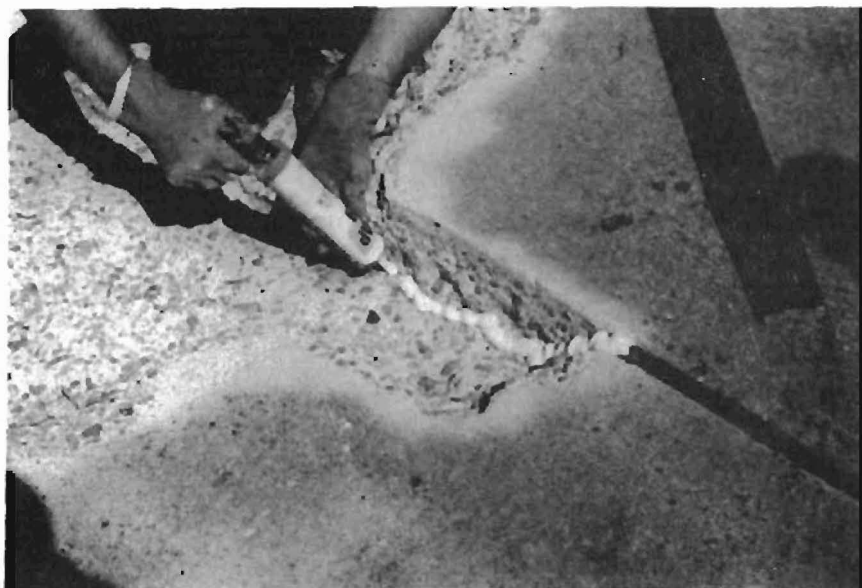
Fig. 4.3 Caulking Joints to Prevent Monomer Leakage.
