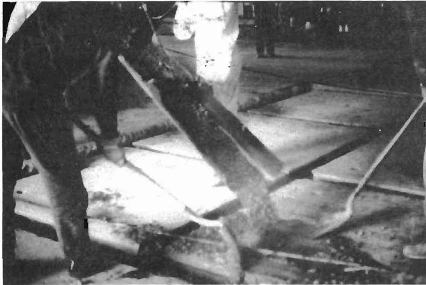
Fig. 4.9 PC Being Discharged from Concrete Mobile ® .
