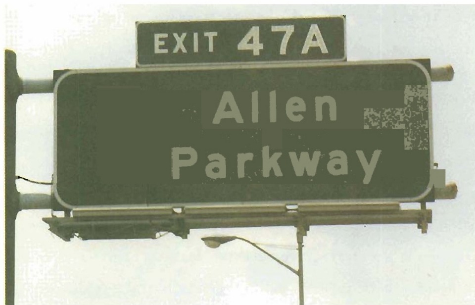
Refurbished Sign Panel using Rigid Aluminum Overlay Coated with High Specific Intensity Reflective Sheeting and High Specific Intensity Stick on Copy
