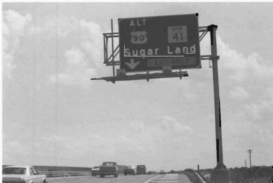
Figure 17: Refurbished Sign Panels using High Specific Intensity Reflective Sheeting Applied Directly to the Aluminum Extrusions after 3 years of service - Good Condition
