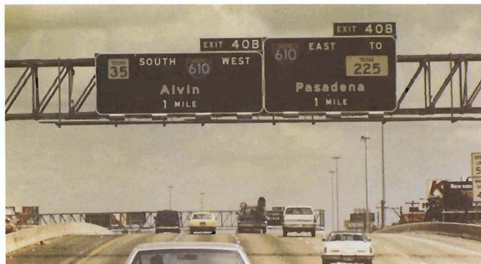
Figure 13: Two Thermal Setting Polyester Coated Sign Panels and 100 Watt Mercury Vapor Sign Lights. This contract installation was made in 1982.
