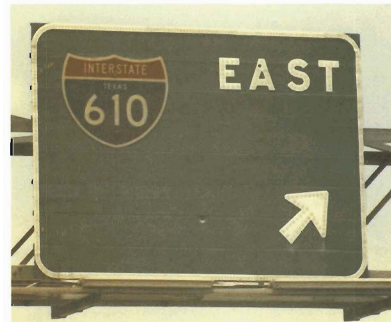
Sign Refurbished with GES-2C Sign Enamel after 7 years Service
