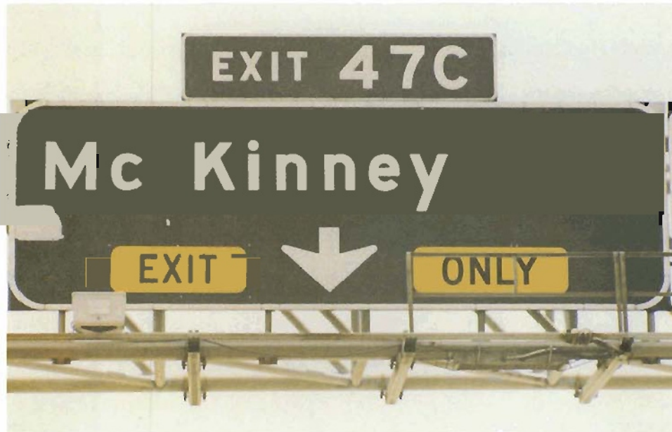
Figure 12: Showing Thermal Setting Polyester Coating Delamination due to Improper Cleaning or Handling of Substrate during Coating Process - Otherwise in Good Condition in regards to Color and Surface Condition
