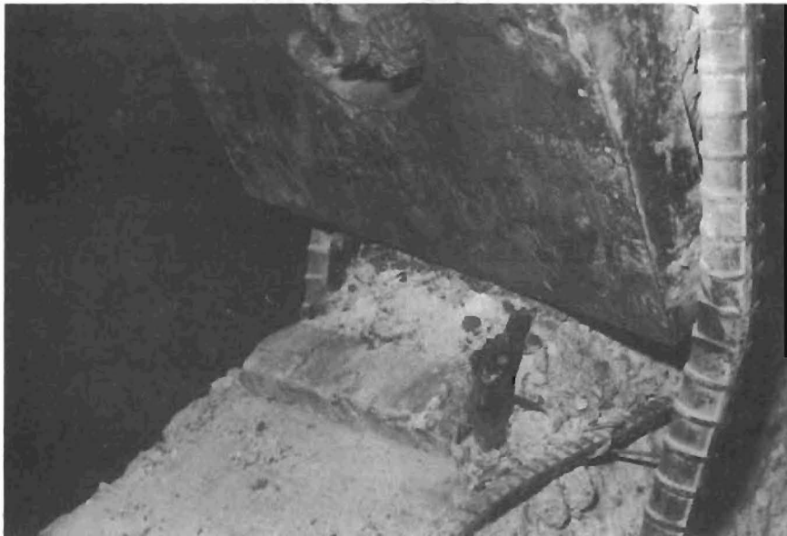
(h) Failure of lateral prestress tendons initiated explosive failure
