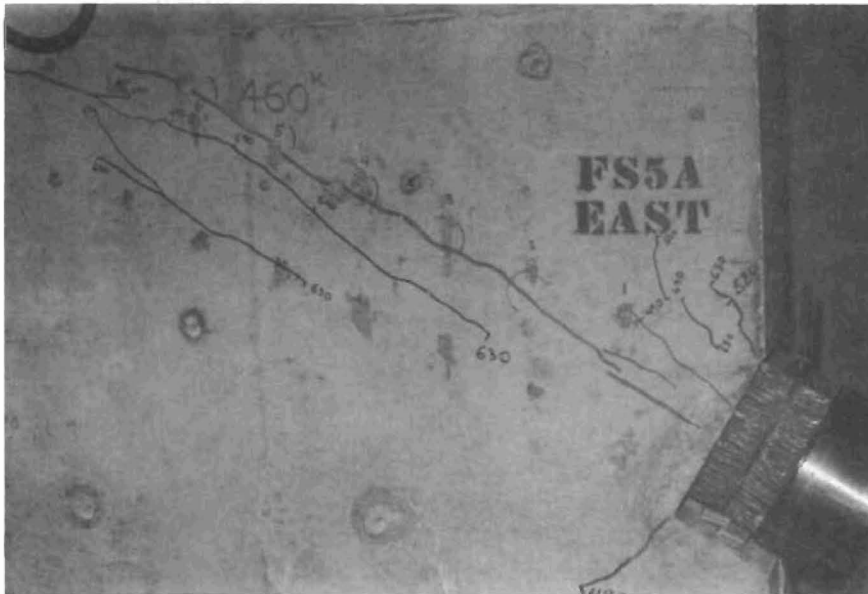
(e) Longitudinal cracks near point of maximum curvature (east side) at 630 kips
