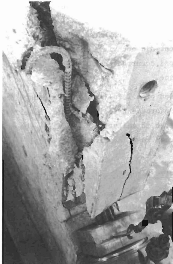
(e) Ultimate load (650 kips) FS4A. Close up of anchorage area
