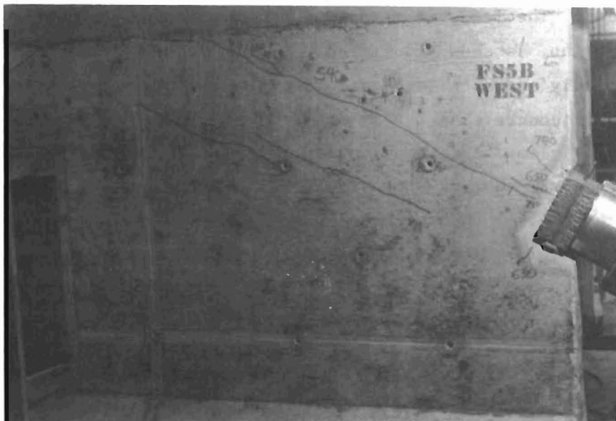
(b) Formation of multiple longitudinal cracks just prior to failure
