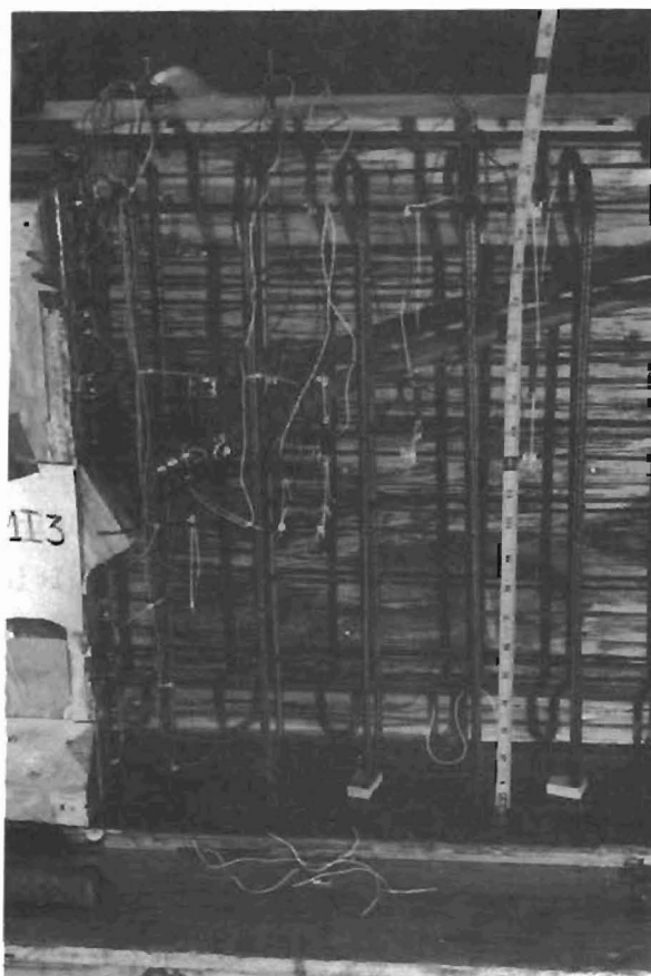
Fig. 4.7 Attachment of curved tendon to end form
