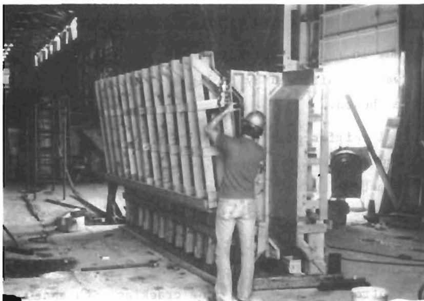
(f) Top of side form lifted into place
