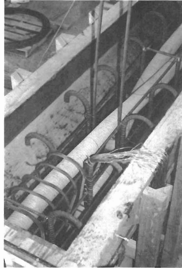
(d) Top view of closed forms showing lateral post-tensioning tendons and primary tendon duct
