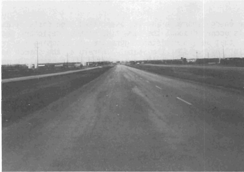
Figure 2 Example of Aggregate Loss in Wheel Paths
