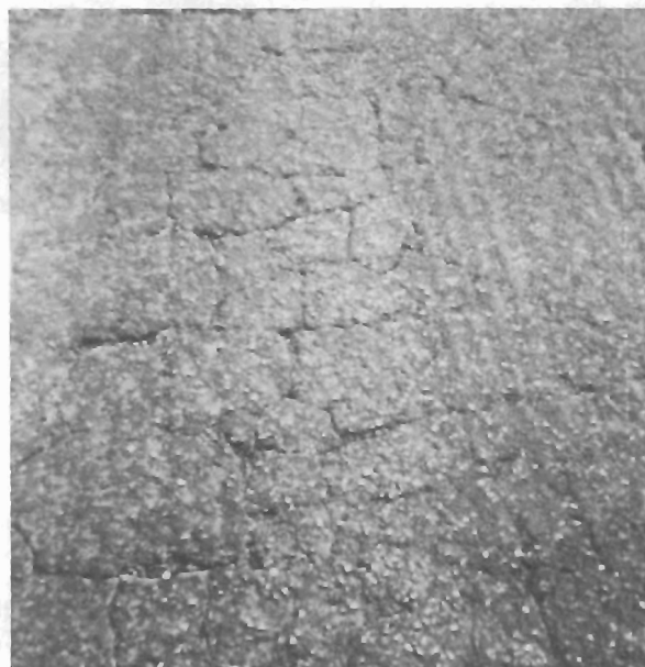
Figure 8 Scarifier Teeth Marks in Pavement
