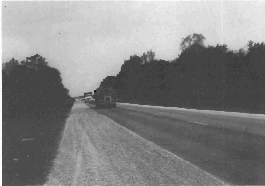
Figure 5 Traffic on Recycled Roadway
