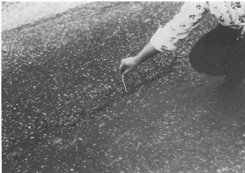
Figure 7 Surface Cracking
