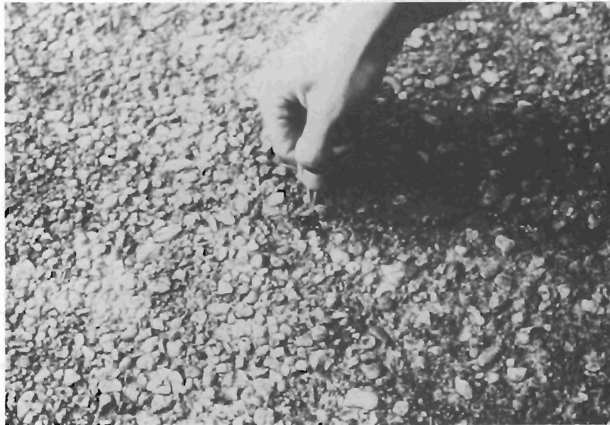
Figure 4 Close-up of Roadway Texture Between Wheel Paths
