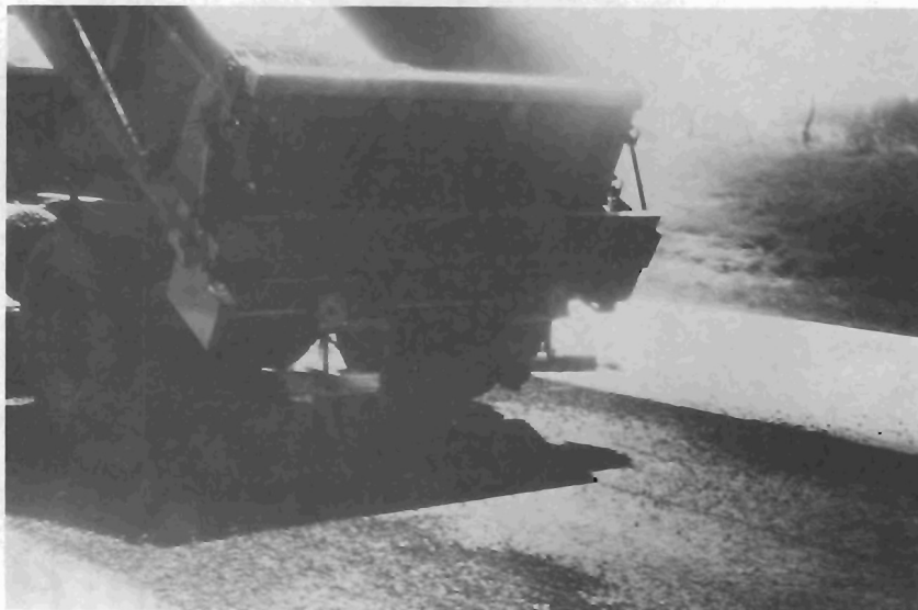
Figure 23 Sprinkle Treatment Application Using Salt Spreaders
