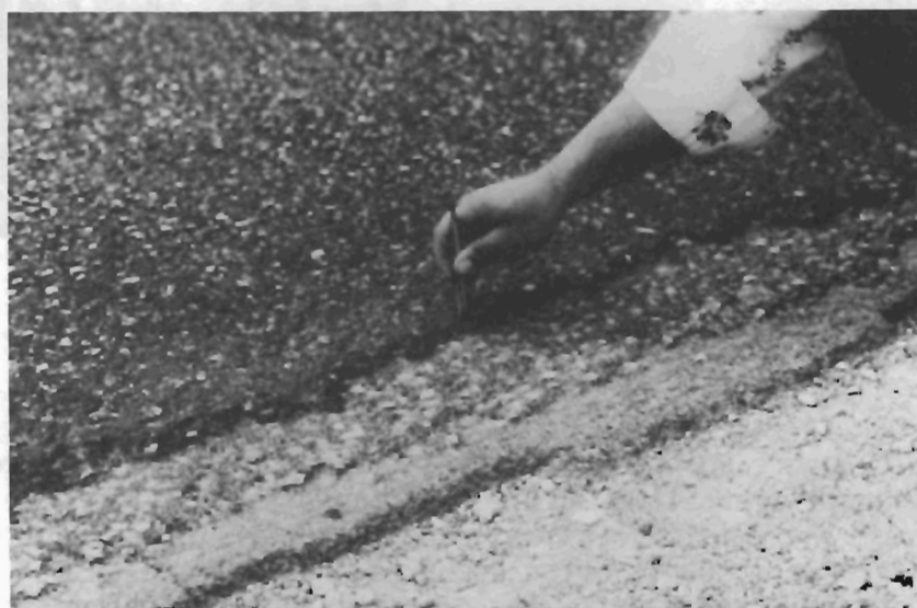
Figure 10 Edge of Recycled Pavement
