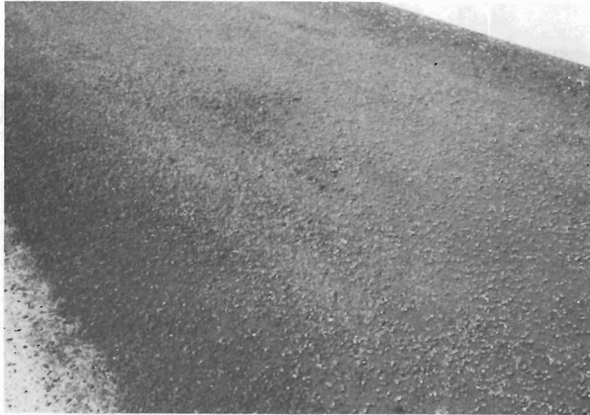
Figure 24 Sprinkle Treated Surface Prior to Rolling
