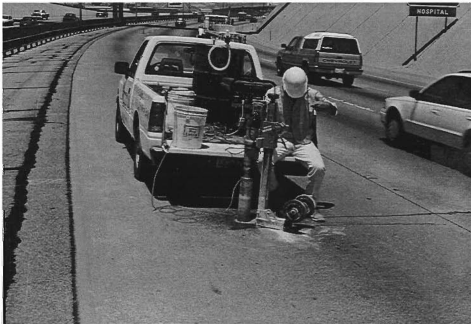
Figure 2.18 Coring on IH-10 westbound
