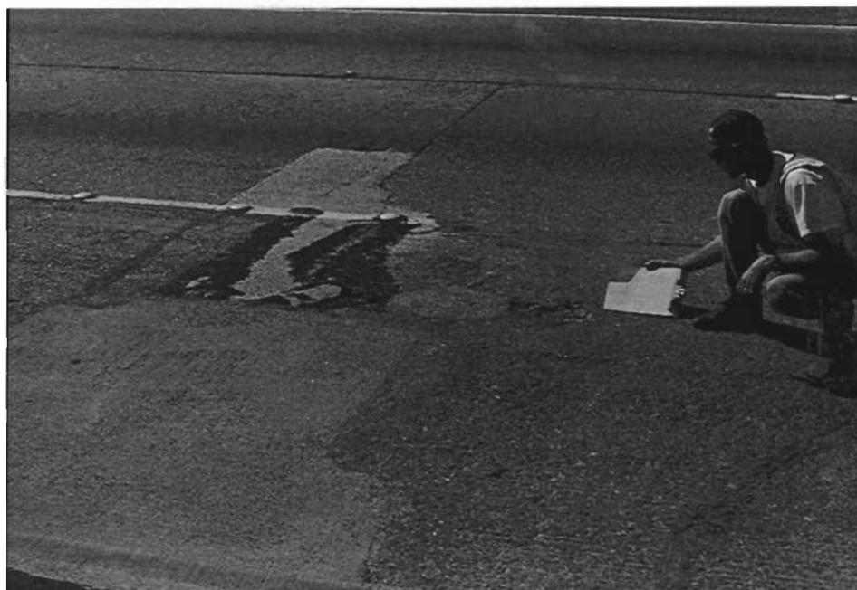
Figure 2.17 Example of popout on IH-10
