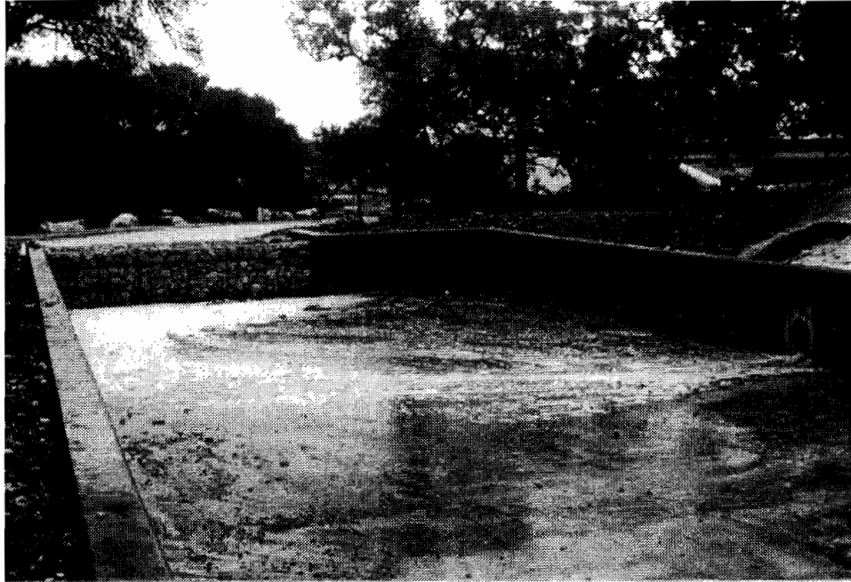
Figure 3.3 Retention Basin Filling with Highway Runoff.
