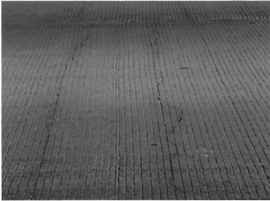
FIGURE 6 Typical CRCP section with 100 % recycled aggregates.
