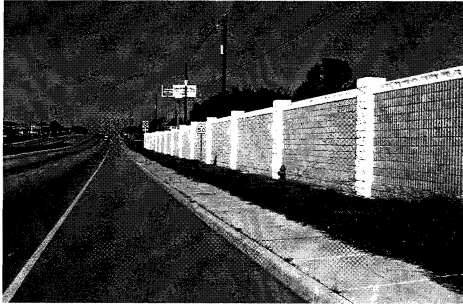
Figure 5.6. Constructed-in-Place Post and Panel System in Austin (reinforced masonry posts and panels)
