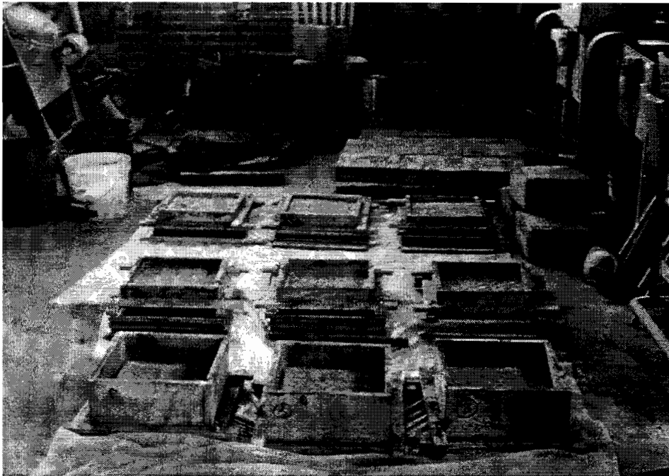
Figure 4.6 Formwork used in casting repair materials
