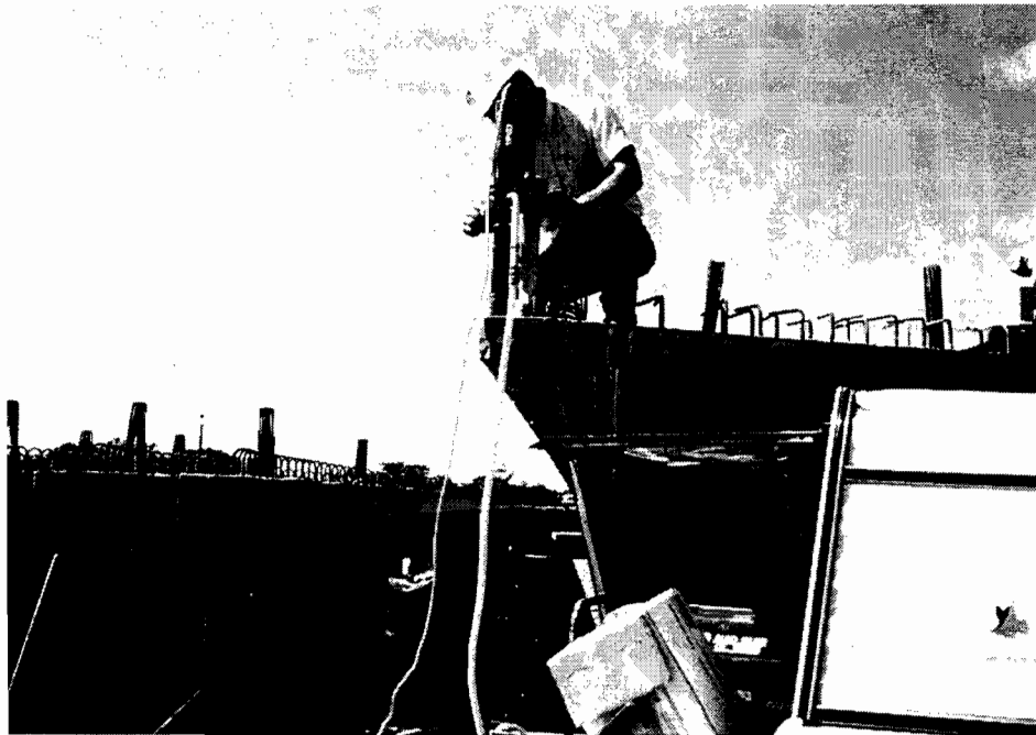
Figure 6.14 Coring repaired corner of U-beam — Victoria No. 6
