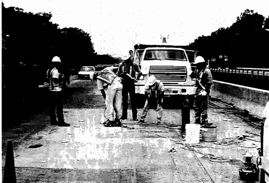
Figure 6.11 Horizontal coring of repaired bridge deck — Lufkin No. 1
