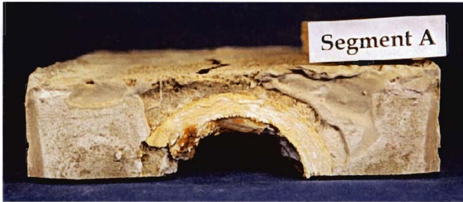
Figure 4.18 – Incomplete Epoxy Coverage in Epoxy/Gasket Joint (EG-S-M-NG-2)
