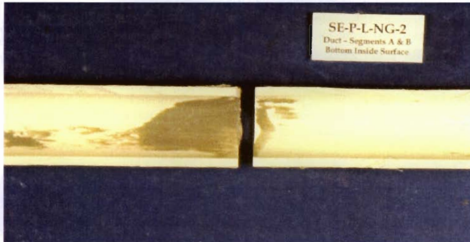
Figure 4.17 – Joint Epoxy Smearred Inside Plastic Duct During Swabbing
