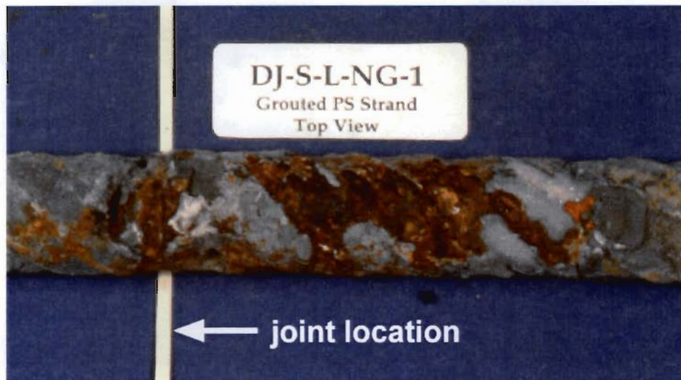
Figure 4.12 – Heavy Rust Staining on Grout Surface
