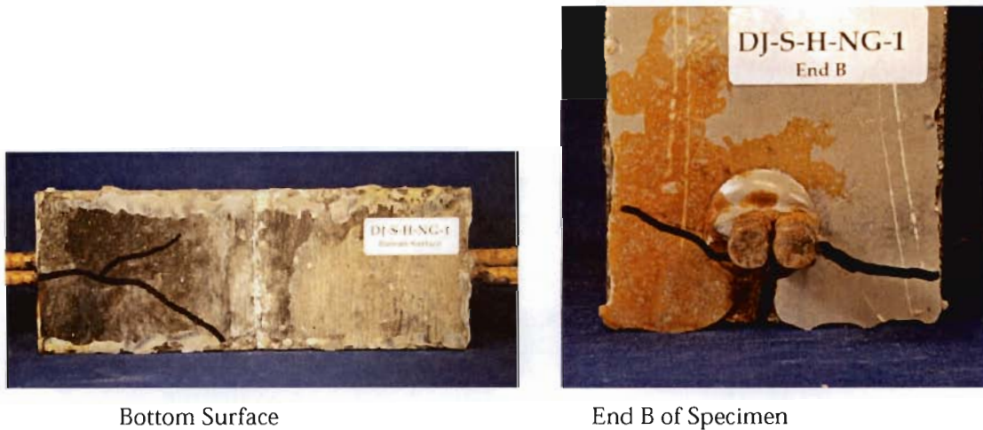
Figure 4.14 - Cracking Due to Rebar Corrosion
