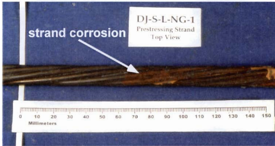
Figure 4.11 – Moderate Prestressing Strand Corrosion Where Epoxy Paint Peeled Away (Segmental Joint Location Indicated by Vertical White Line)
