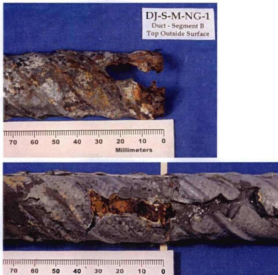
Figure 5.6 - Hole in Duct Corresponding to Grout Void
