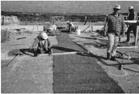
c). Deck joint concreting
