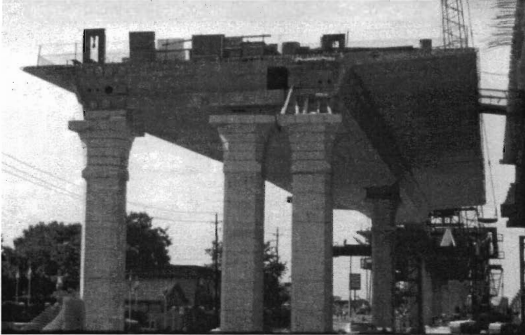
Figure 1.9 Cast-in-place transition spans
