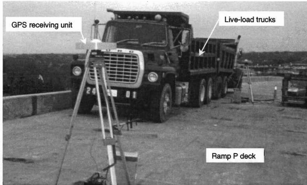
Figure 2.29 GPS deflection measurement equipment
