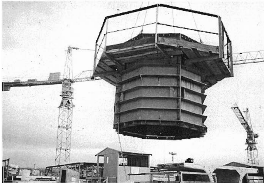
Figure 1.37 Placement of outer pier segment form
