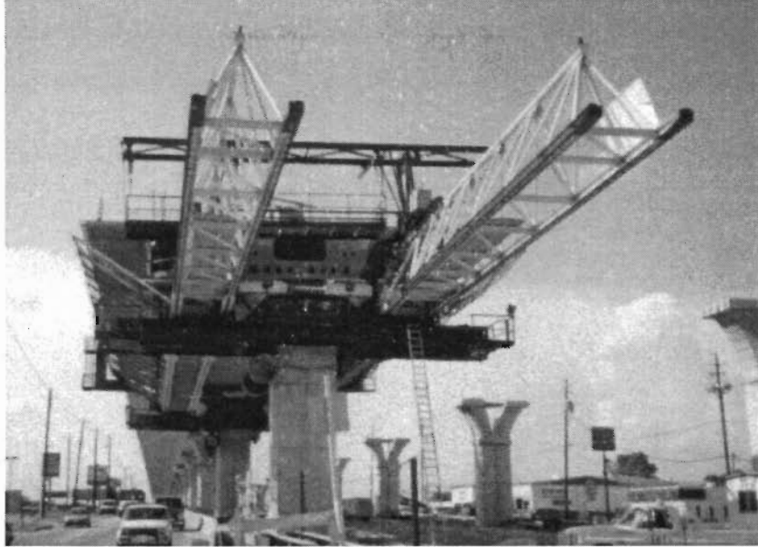
Figure 1.18 Construction of a mainlane girder
