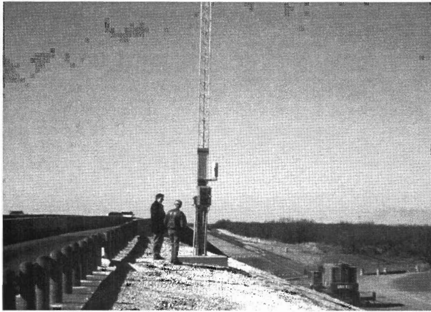
Figure 3.5 RPU tower installed near Abilene
