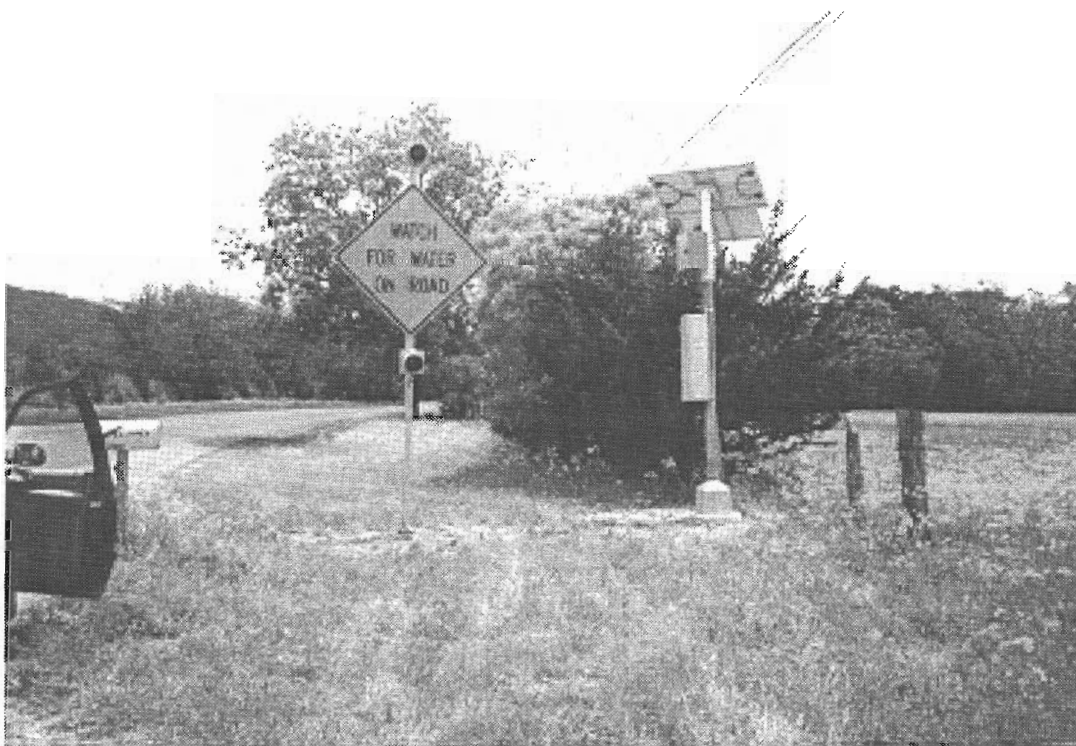
Figure 3.2 Sign complemented with flashing lights
