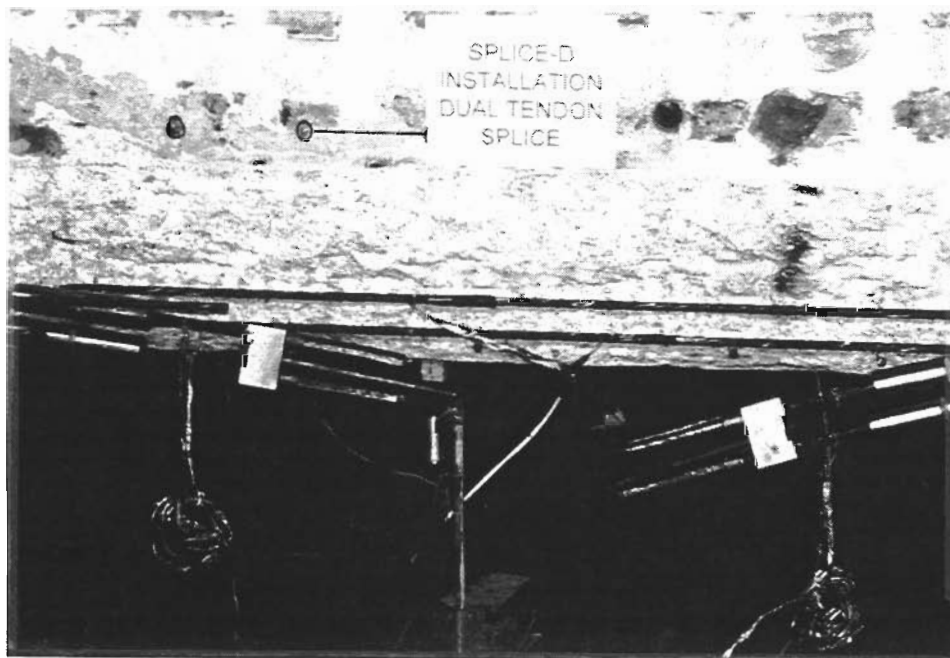
Figure 6- 43 Installation of dual strand swaged splice assembly
