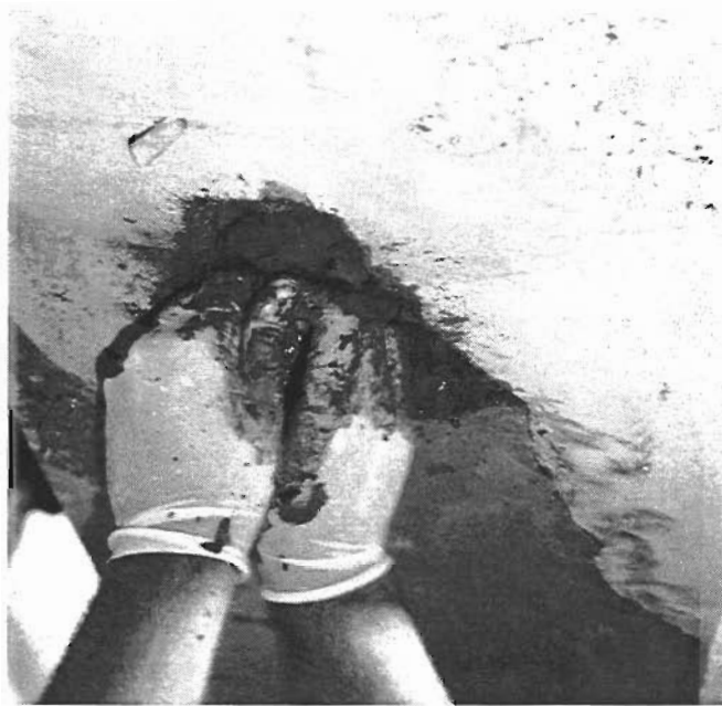
Figure 5- 20 Overhead repair of bottom flange using Burke V/O
