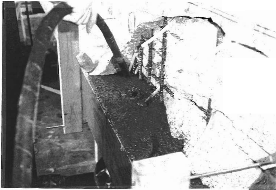
Figure 5- 13 Placement and consolidation of Patchroc 10-61
