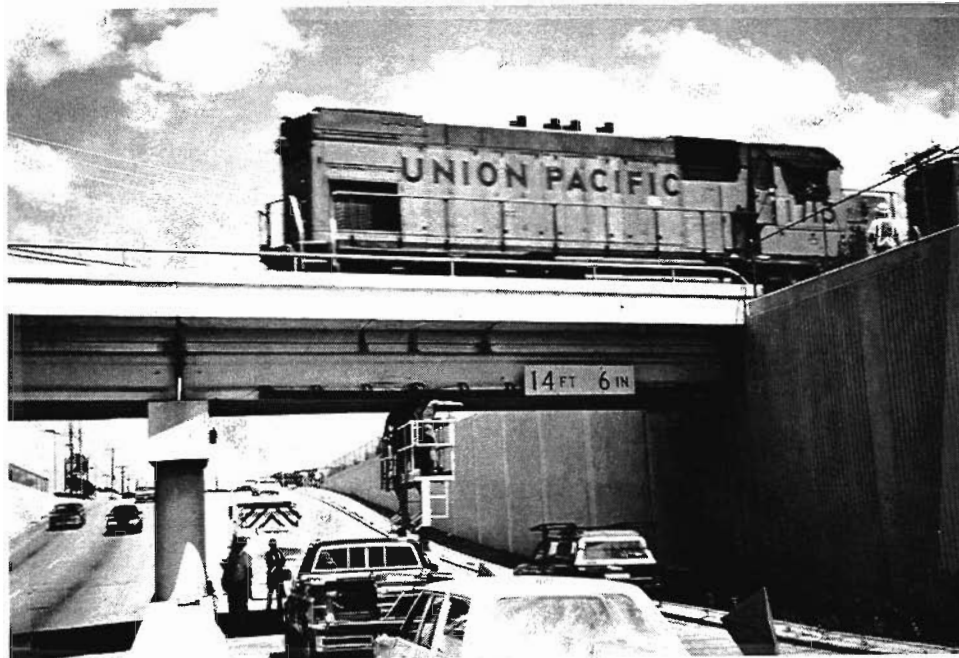
Figure 4- 2 Overall view of Steck girder in-situ
