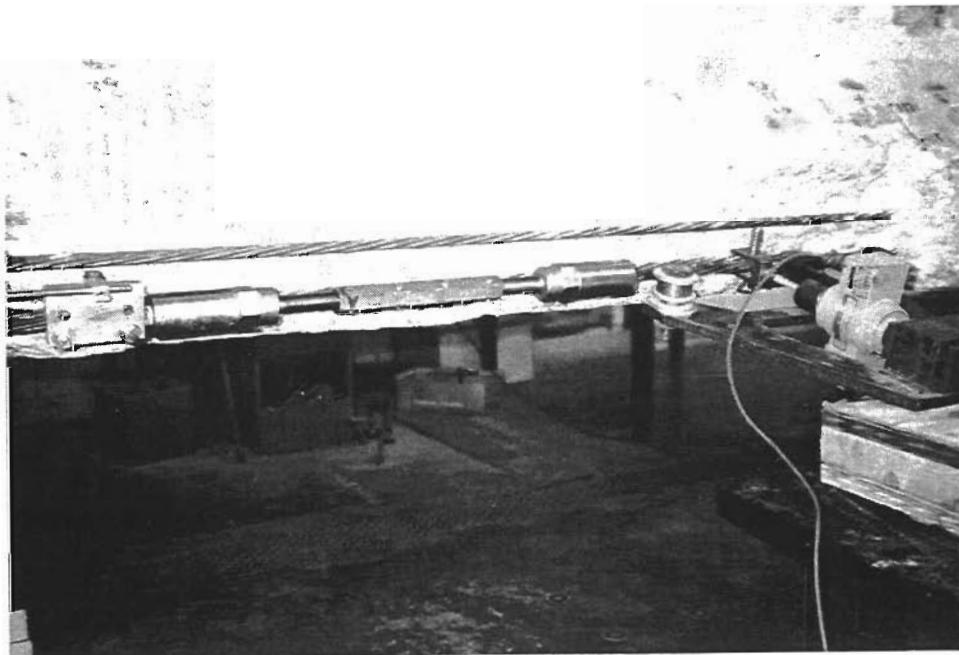
Figure 6- 53 Completed installation of the Grab-It™ splice
