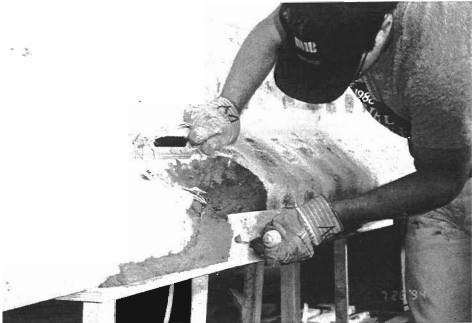
Figure 5- 17 Partially formed bottom flange repair using Renderoc HB2
