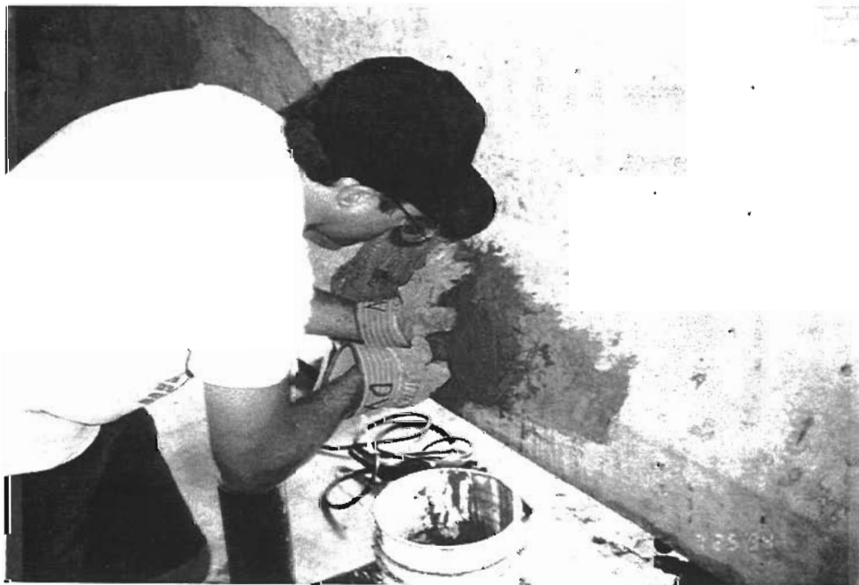
Figure 5- 19 Repair of the bottom flange on the nonimpacted face of girder using Burke V/O
