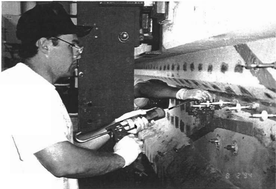
Figure 5- 23 Epoxy injection using low pressure injection system
