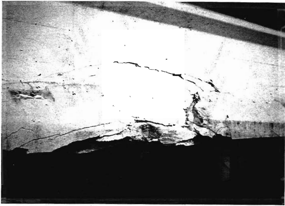
Figure 4-4 Close-up view of Steck girder after removal — direct area of impact
