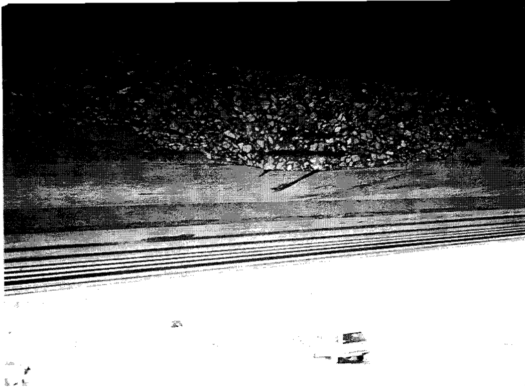
Figure 5-6 Loss of side cover example (Courtesy of Texas Department of Transportation)
