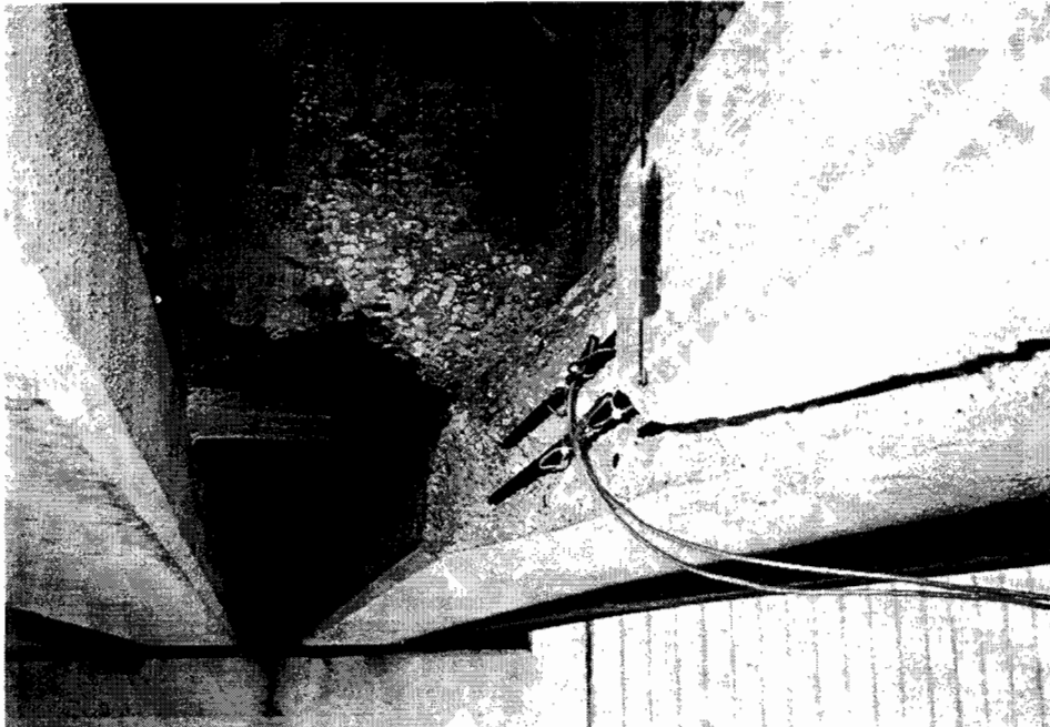
Figure 5- 12 Instrumentation of exterior girder
