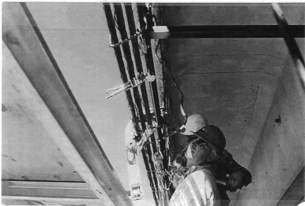
Figure 5- 15 Retensioning operation of severed strands
