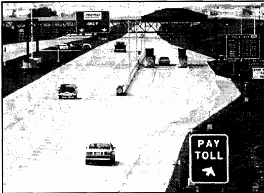
Figure 7.1. An Example of Free Flowing Lanes (from "The PIKEPASS Connection Oklahoma Motorists Avoid Tollbooths." Government Technology, August 1992)
