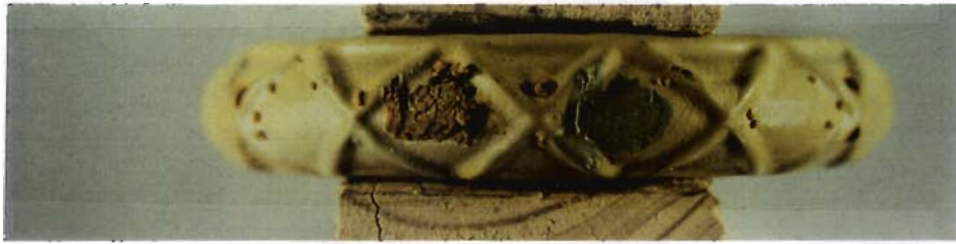
Figure 5.3 Deterioration of exposed areas and holidays on #4 bar with cross deformations.
