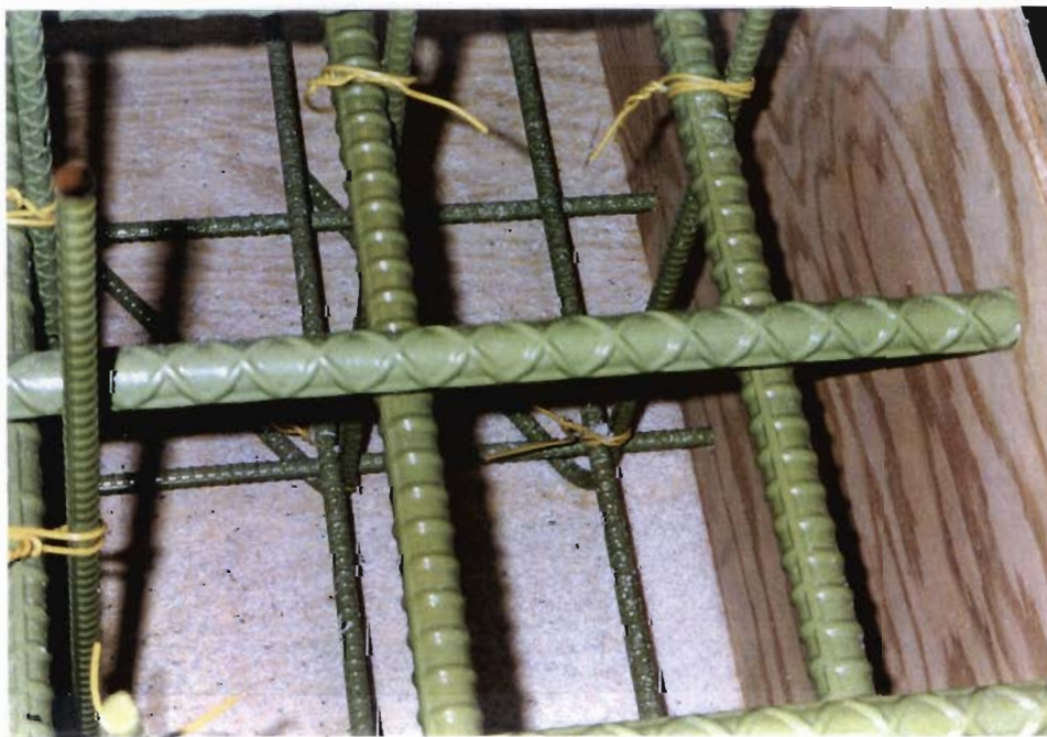
Figure 4.3 Plastic-covered wire used to tie reinforcement.
