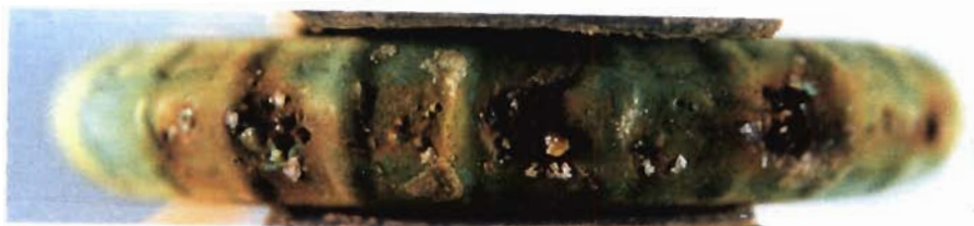
(a) Corrosion in patched areas
