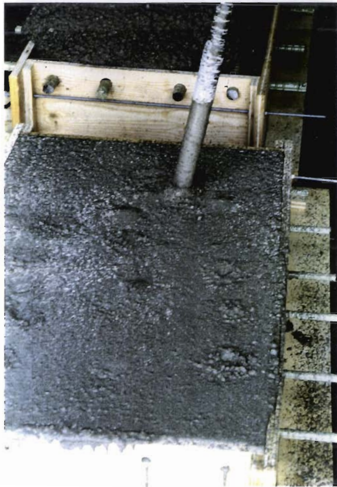
Figure 4.9 Vibration of the slab specimens.
