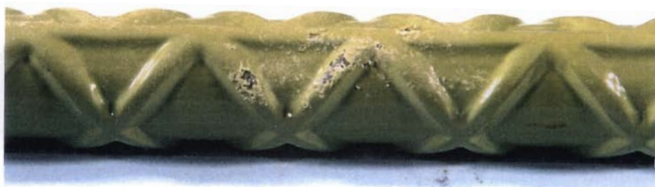
Figure 4.12 Damage due to vibration on the bottom side bars in the column specimen.
