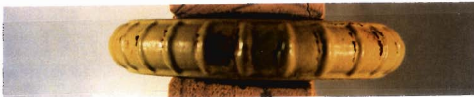
Figure 5.2 Deterioration of exposed areas on #4 bar with parallel deformations.
