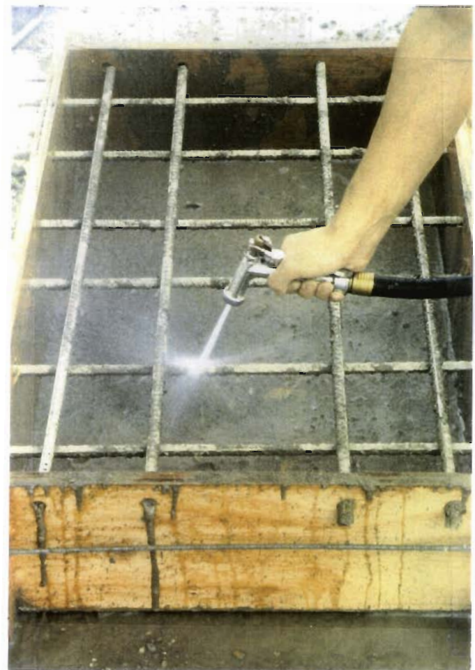
Figure 4.10 Washing the bars after concrete removal.
