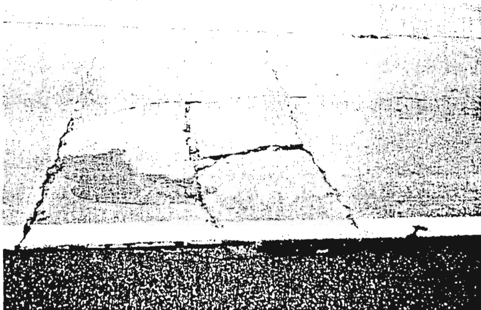
Figure 2.16.2: IH-45 Test Section in Buffalo, Punchout
