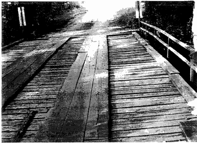
Figure 5.15 Bastrop County Bridge AA-0237-01.
