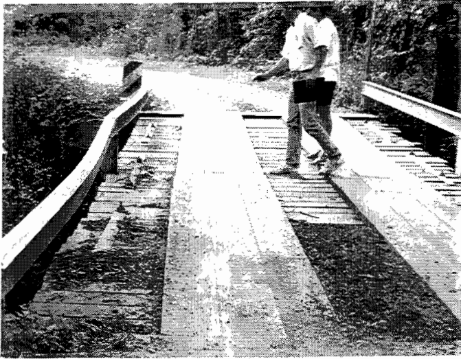
Figure 5.14 Bastrop County Bridge AA-0233-01.
