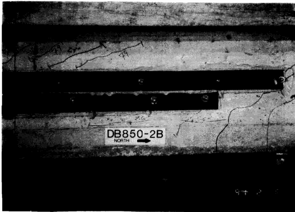
Figure 5.6 Bursting Crack Developed During Test DB850-2B (S)
