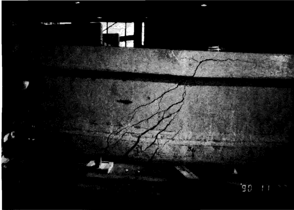
Figure 4.30 Web Shear Cracking, DB850-1A (G)
