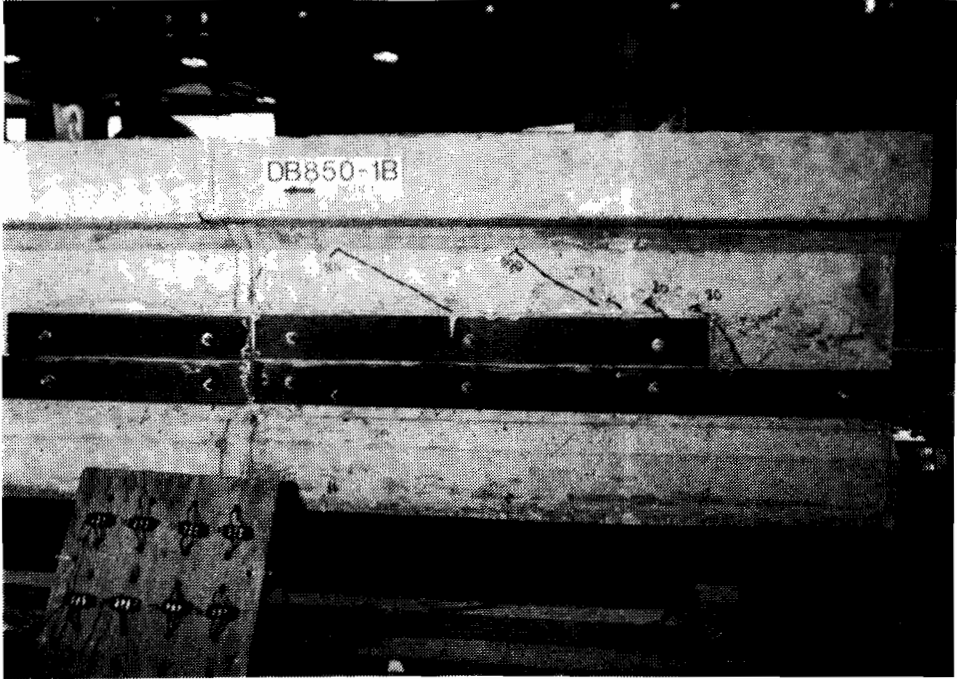
Figure 5.4 Web Shear Cracking in Debond/Transfer Zone
