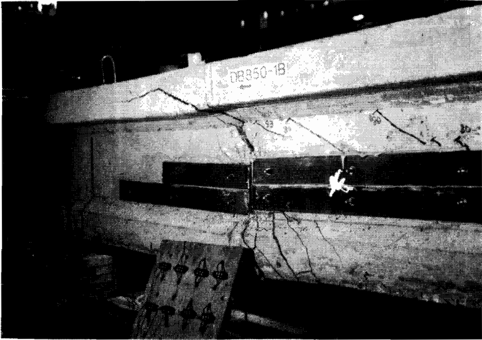
Figure 5.5 specimen Collapse from Web Shear Cracking
