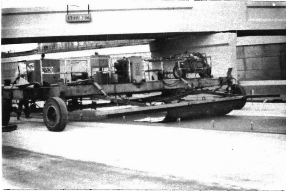
Fig 3.2. Mechanical texturing of pavement in the field.
