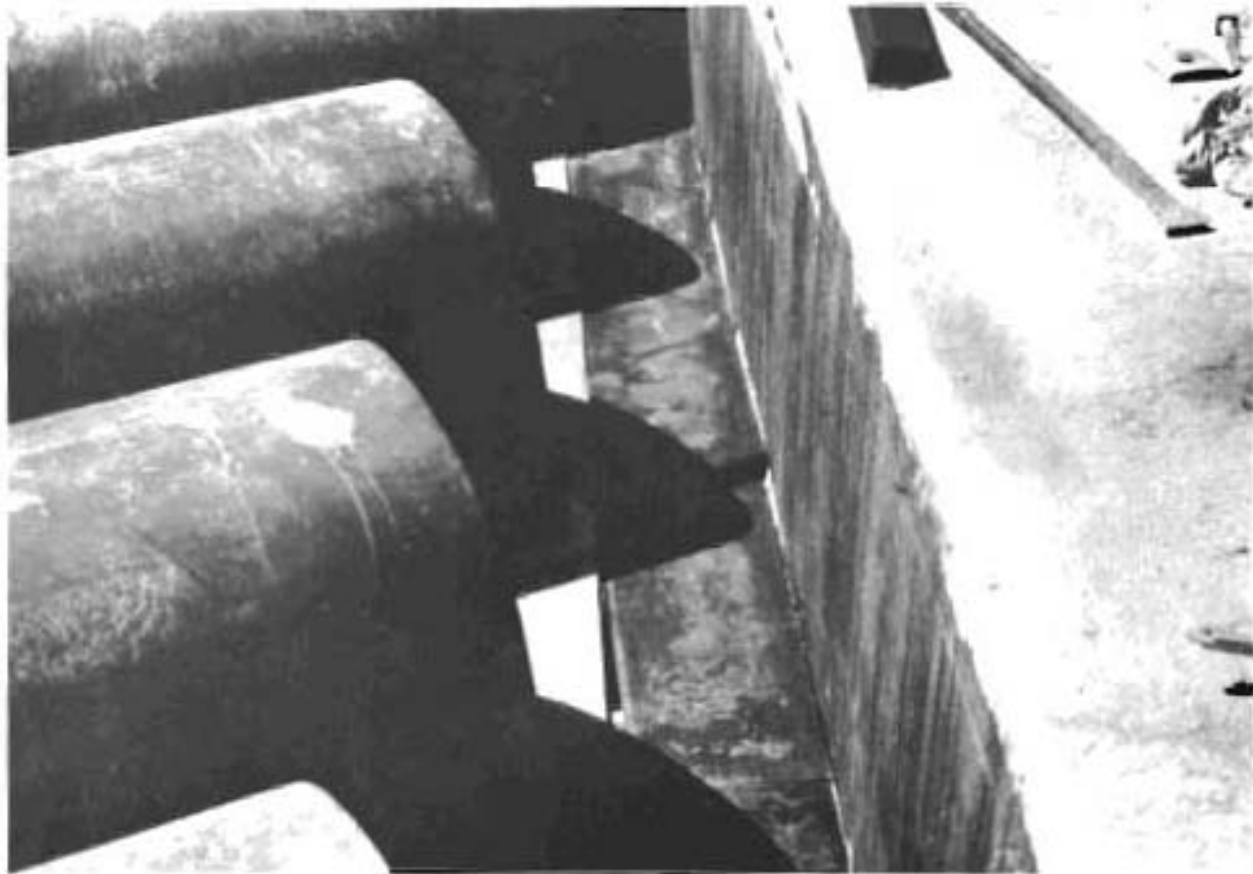
Fig. 1.4. Pan Form Support Details.
