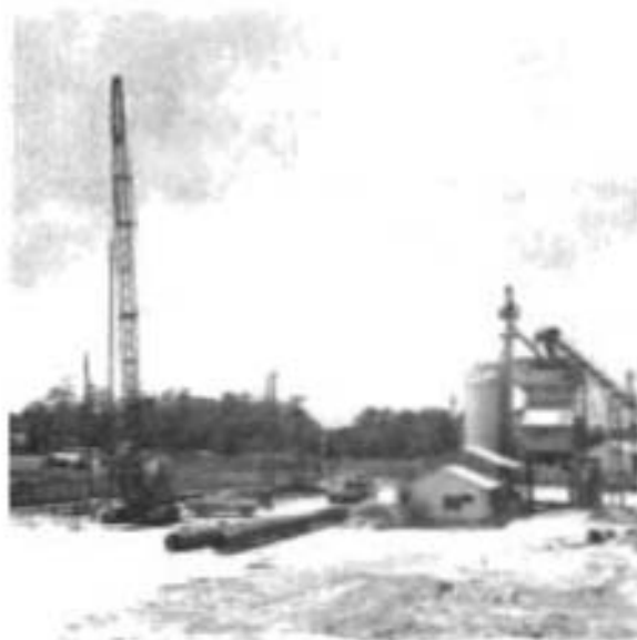
Fig. 5.3. Drilling Rig Working at the HB&T Test Site
