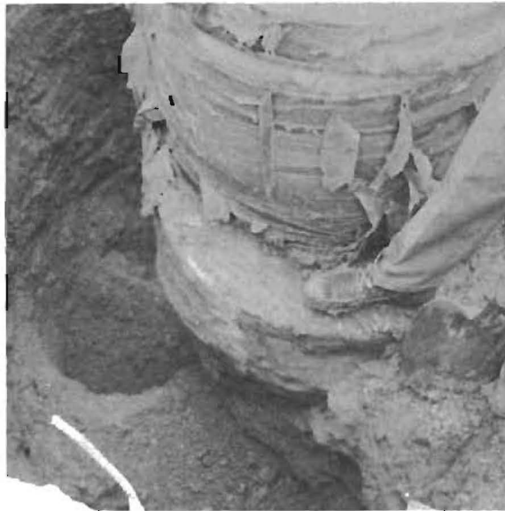
Fig. 6.5. Shaft Enlargement in Upper Section
