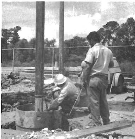
Fig. 5.5. Setting of Casing for the HB&T Test Site
