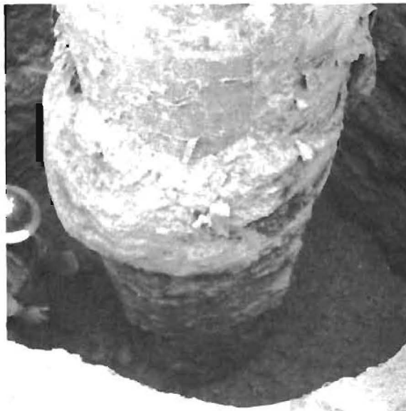
Fig. 6.6. View of the Test Shaft from Ground Surface to Approximately the 13 Foot Level
