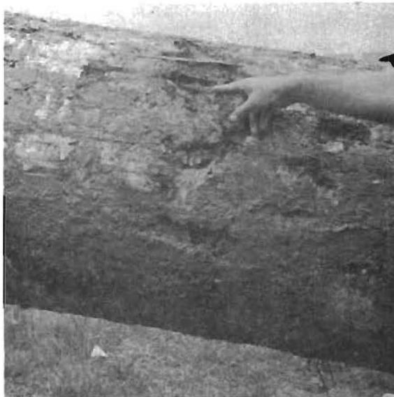
Fig. 12.75. View of Honeycombed Section
