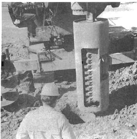
b. Belling Tool in Closed Position for Lowering into Borehole
