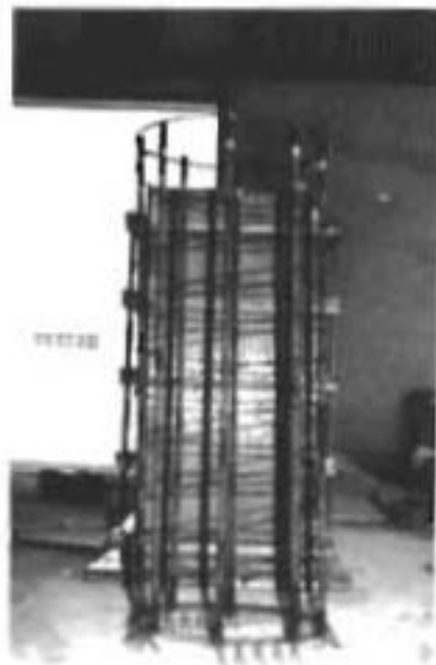
Fig. 7. Form and cage
