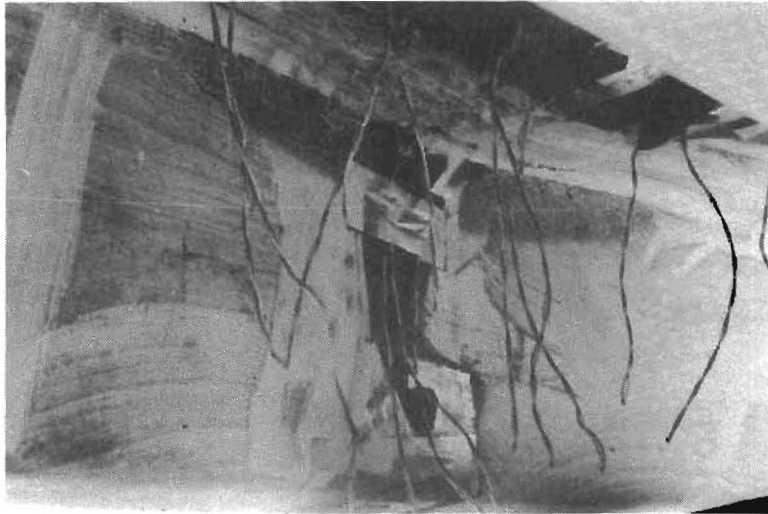
Buckling of Rib Inner Wall Flanged Specimen
