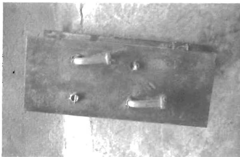
FIGURE 10. TYPICAL STUD FATIGUE FAILURES IN STEM OF STUD
