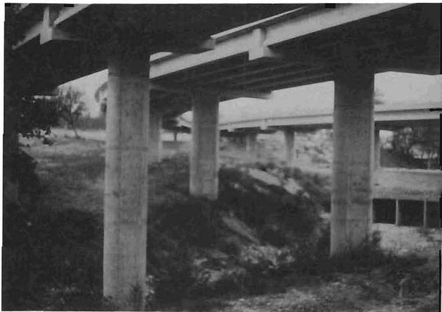
Fig. 1.1. Part circle support: Interstate 35, Austin, Texas.
