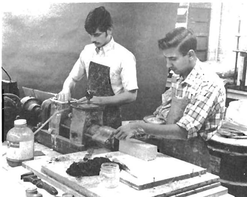
Fig 5. Extrusion of soil in the form of prismatic block.
