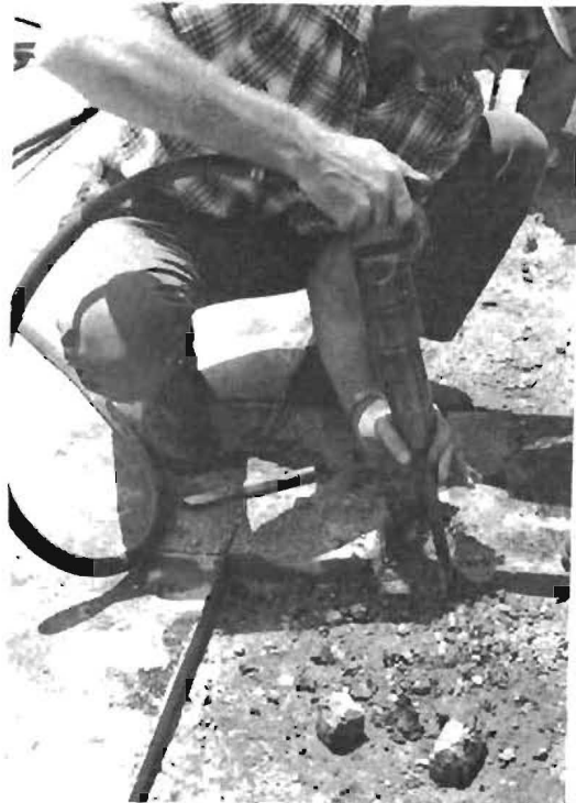
Fig B.2. Removal of pavement.
