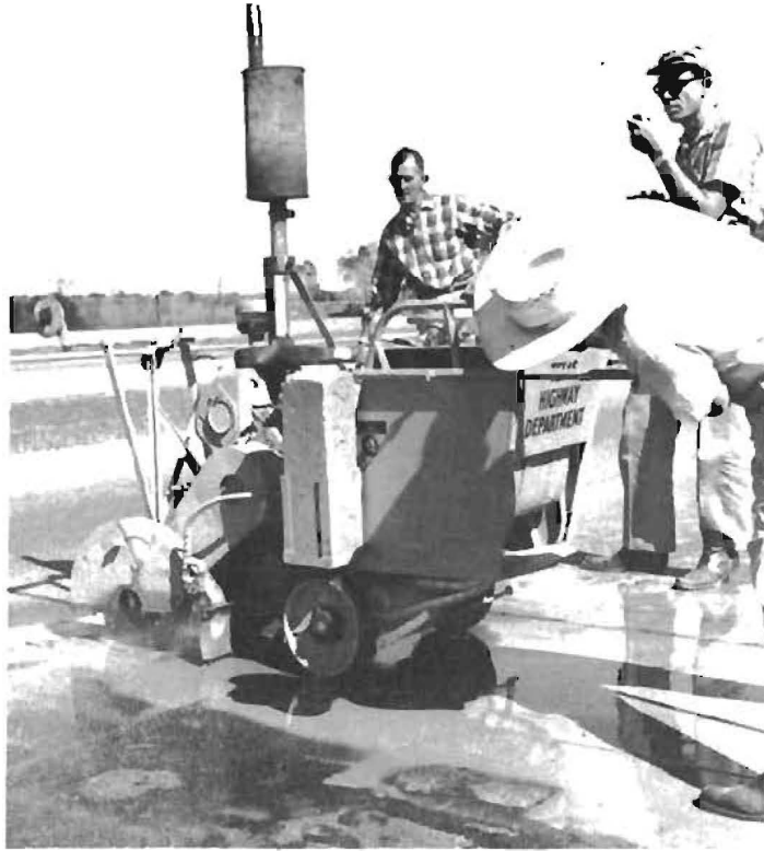
Fig B.1. Saw cutting operation.
