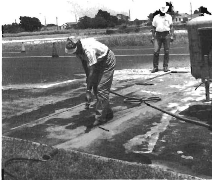
Fig B.3. Saw cuts cleaning.
