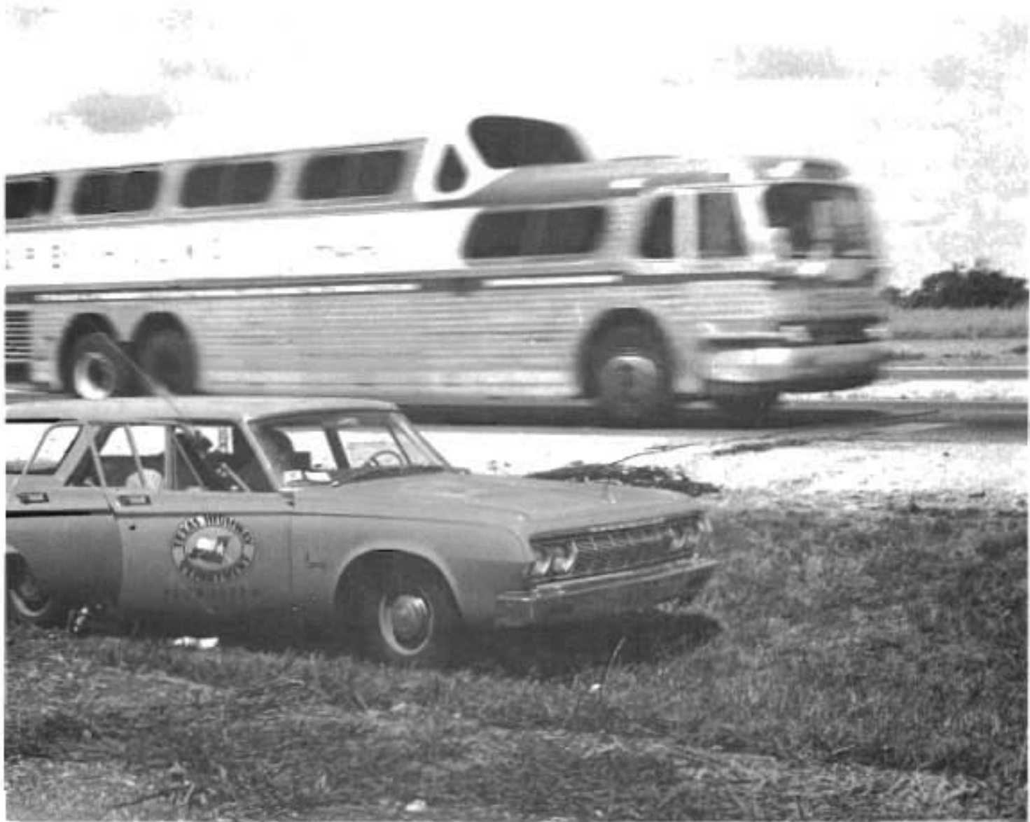
Fig 5.1. Portable scale installation on Interstate 35 at Temple-Belton, Texas.
