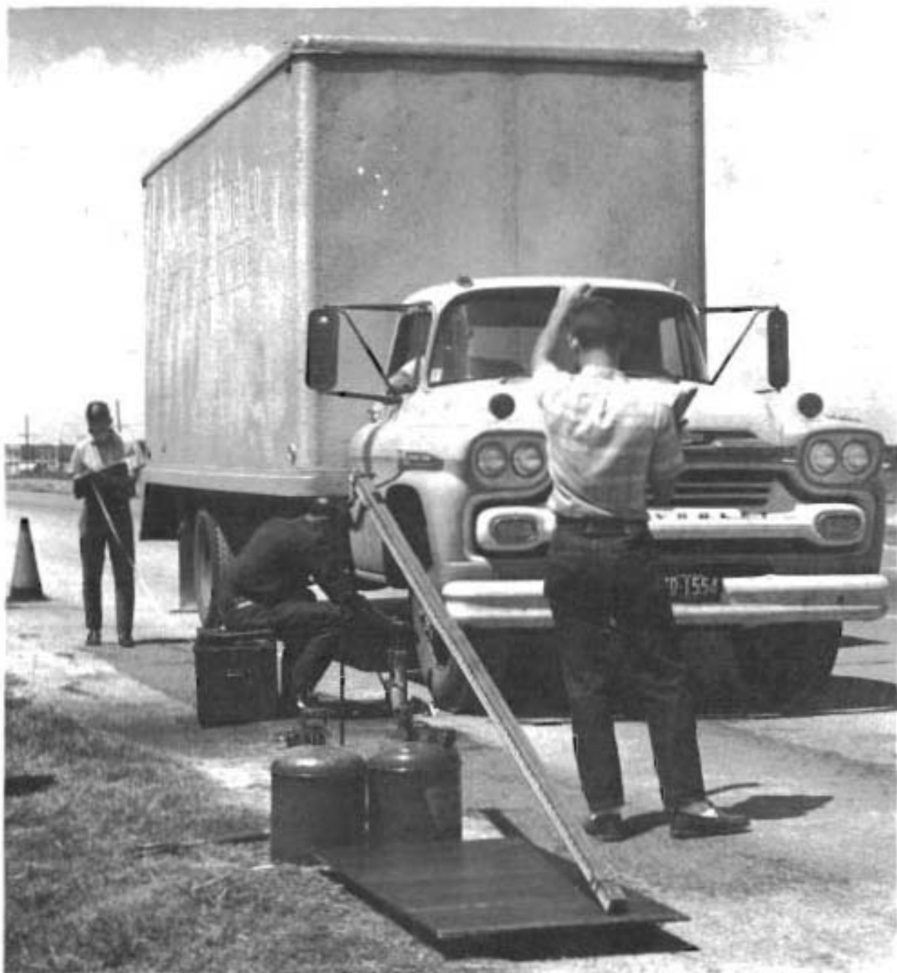
Fig 1.1. Loadometer Station (tire on scale).
