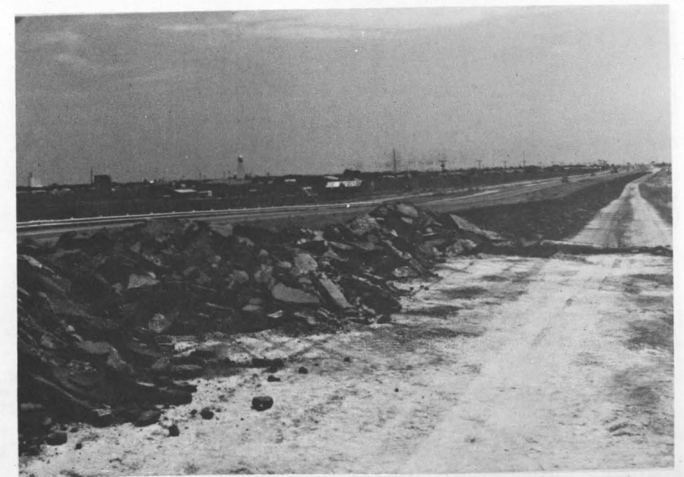
Picture #2 - Scarified material bladed into a windrow.
