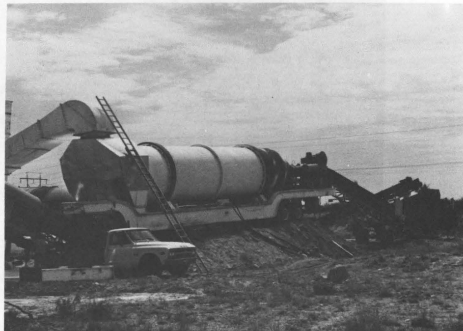
Picture #4 - Modified Boeing Drum-Dryer Plant
