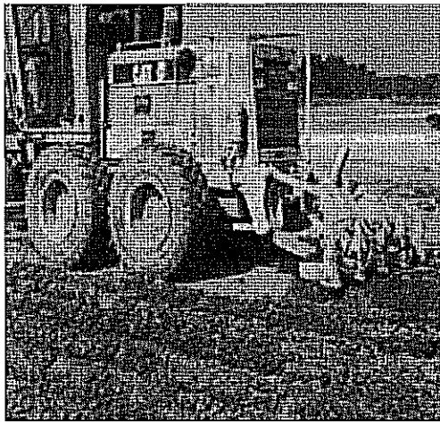
a) Scarification of base material ( www.lime.org )
