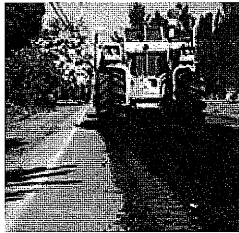
b) Pulverization of asphalt and base ( www.cement.org )
