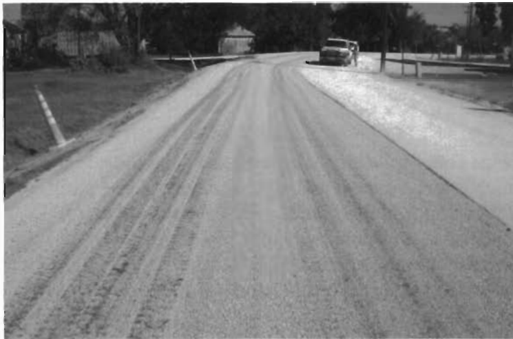
Figure 3.4 Covered (or inverted) prime using RC-250 and grade 5 rock
