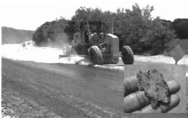
Figure 3.3 Application of worked-in (cut-in) prime on limestone base
