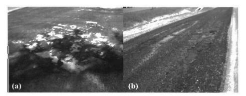
**Figure 13** (a) Prime Peeled-Off at Shaded Area due to Construction Traffic (b) Failed Surface Treatment due to Construction Traffic when Prime Application Base Is Too Wet The "worked-in" prime coat layer is strong enough to run traffic for several days when applied under the 'right' circumstances which are given below:
