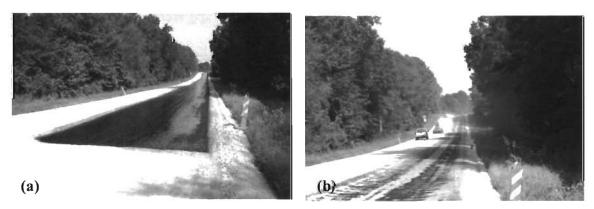
Figure 6 Spray Prime (a) MC-30 Cutback Prime (b) Blotting Sand Applied on Prime
