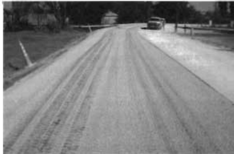
Figure 8 Covered (or inverted) Prime Using RC-250 and Grade 5 Rock
