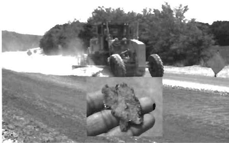
Figure 7 Application of Worked-in (cut-in) Prime on Limestone Base
