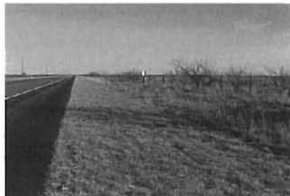
View looking east.
