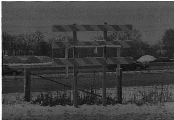
Figure 2-2 Type III Barricade Traffic Gate (Stored Position)
