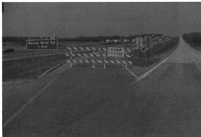
Figure 2-3 Type III Barricade Traffic Gate (Deployed)
