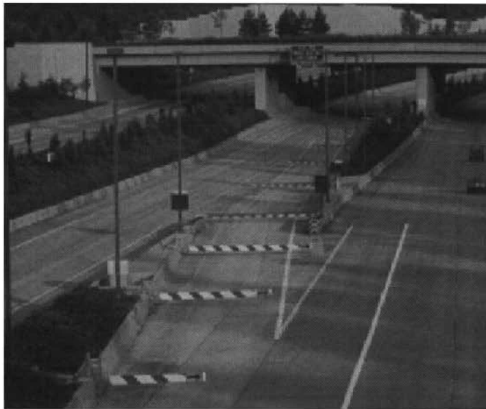
Figure 2-4 Horizontal swing gate( Chicago)
