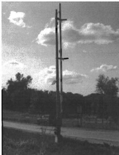
Figure 2-5 Vertical Swing Arm Traffic Gate (Open Position), ITS Design Manual, Wisconsin DOT
