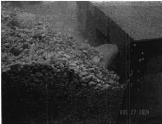
Figure 10. Gravel bed filling culvert.
