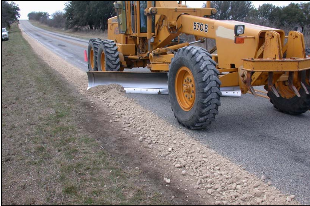
FIG. 5.32 Flex Base for Pavement Edge Repair, Brownwood District, (see Brownwood District Profile, Photograph 15)
