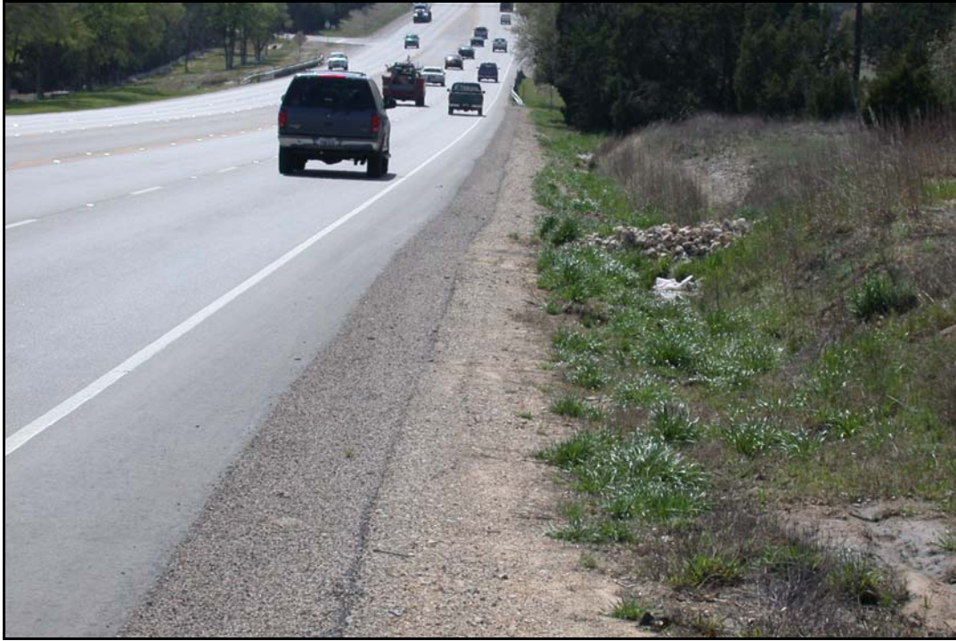
FIG. 5.29 Strip Seal Coat on a Contract Replenishing Project Using Flex Base, Austin District (see Austin District Profile, Photograph 4)
