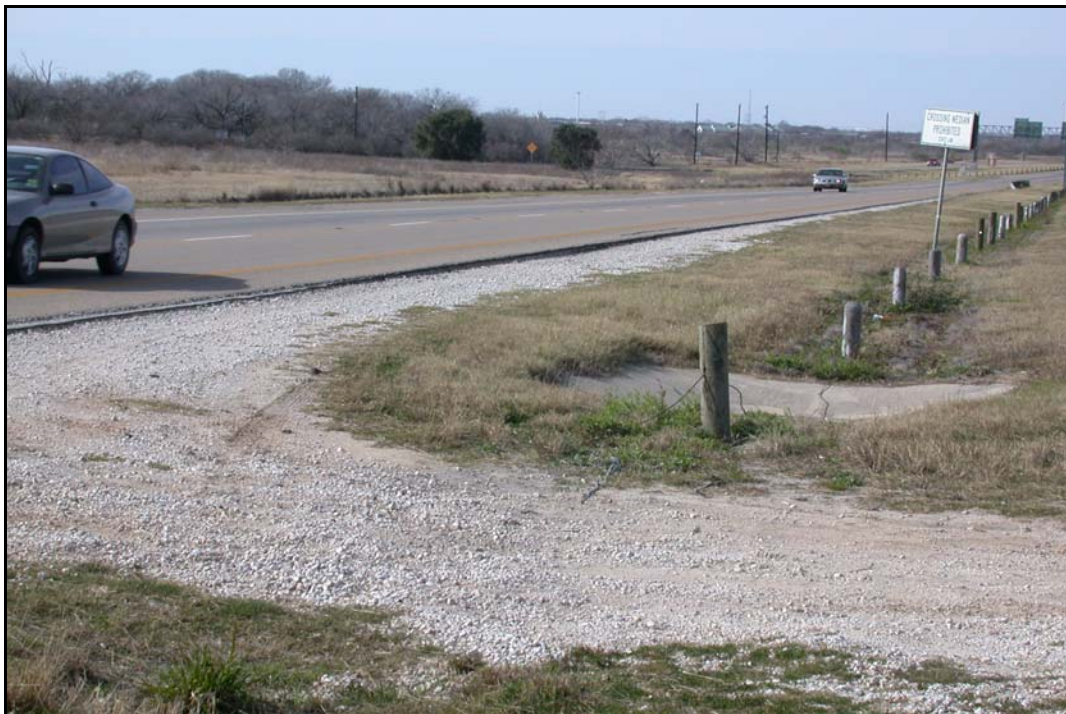
FIG 5.16 Post and Cable Median Barrier, San Antonio District (see San Antonio District Profile, Photo 15)
