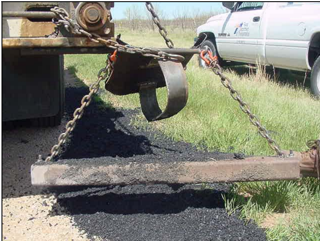
FIG. 7.16 Close-up View, Side Discharge Chute and Tow-Behind Drag Bar for Edge Repair, Wichita Falls District
