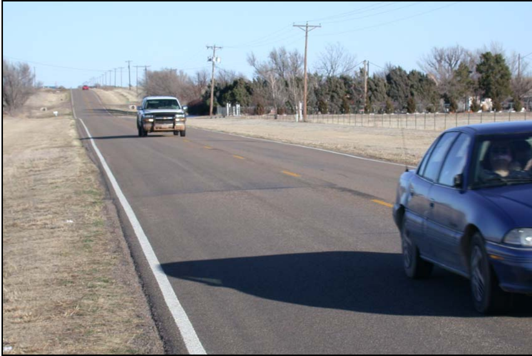
FIG. 6.15. FM 1151 Road Widening, Armstrong County Texas, Amarillo District (see Amarillo District Profile, Photo 29)
