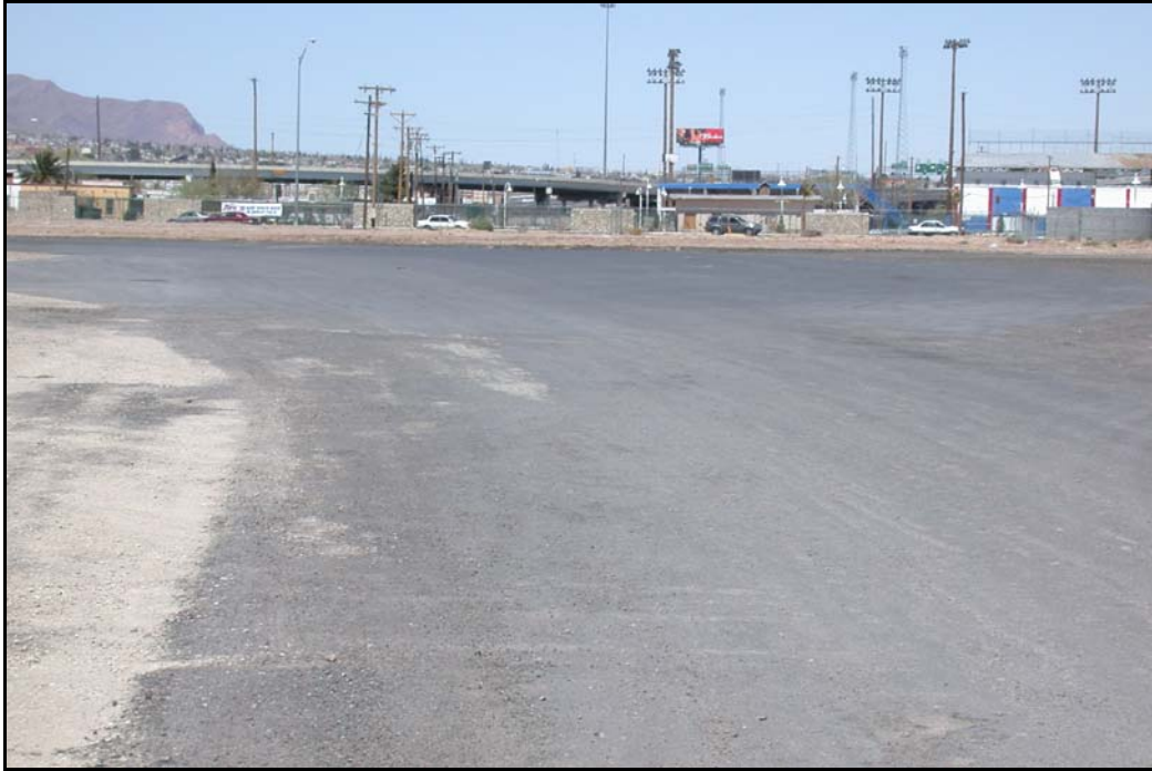
FIG. 5.31 US Customs Truck Parking Lot, RAP Treated with Magnesium Chloride, El Paso District, (see El Paso District Profile, Photograph 23)
