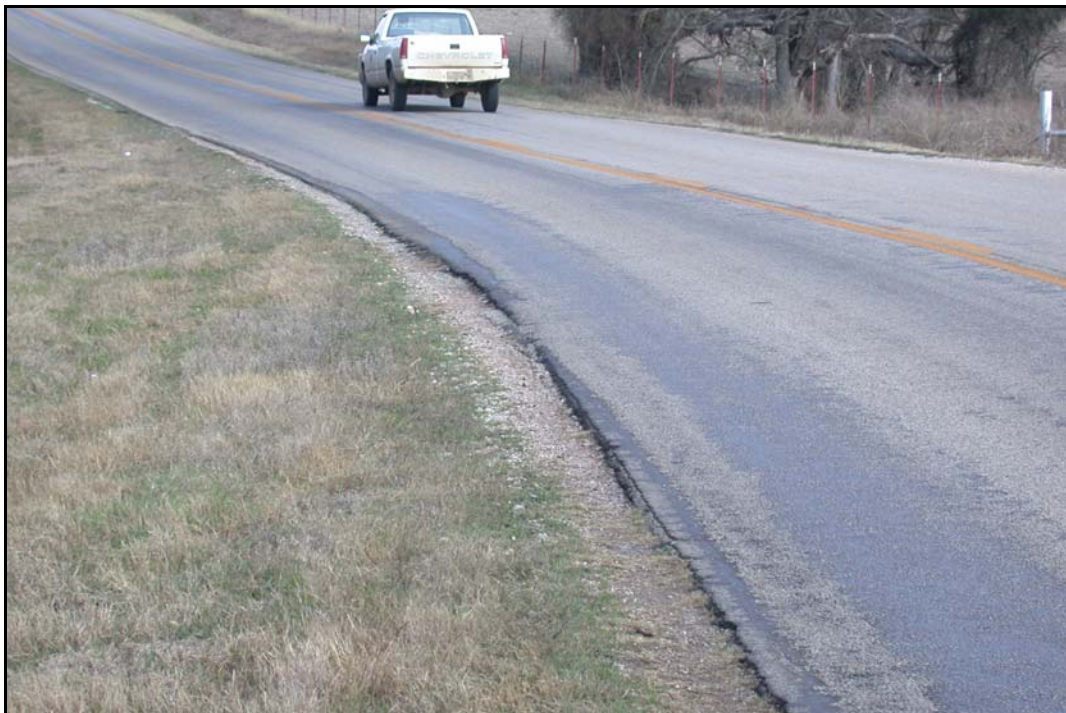
FIG. 4.11. Typical Edge Drop-off at Inside Horizontal Curve on a Low Volume FM Road.
