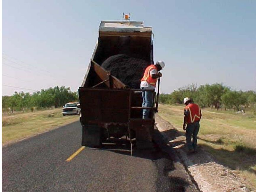
FIG. 7.13 Plywood Insert in Dump Truck Bed to Direct Flow of Material to Side-Discharge Chute, Abilene District ( Photo courtesy of Jones County Maintenance )
