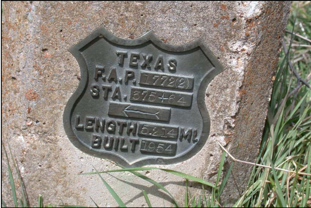
FIG. 4.3. FM Road ROW Marker, Illustrating the Age of the Road (and the System)
