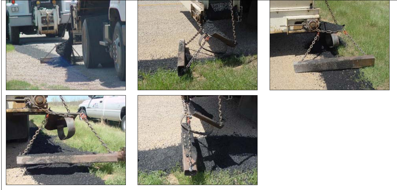
FIG. 7.15 Photo Series: Side Discharge Chute and Tow-Behind Drag Bar for Edge Repair, Wichita Falls District
