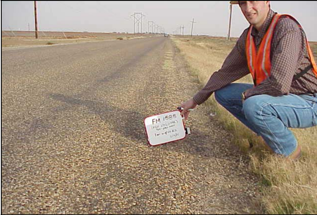
FIG. 6.17. FM 1585 Road Widening, Lubbock County Texas, Lubbock District (see Lubbock District Profile, Photo 13)
