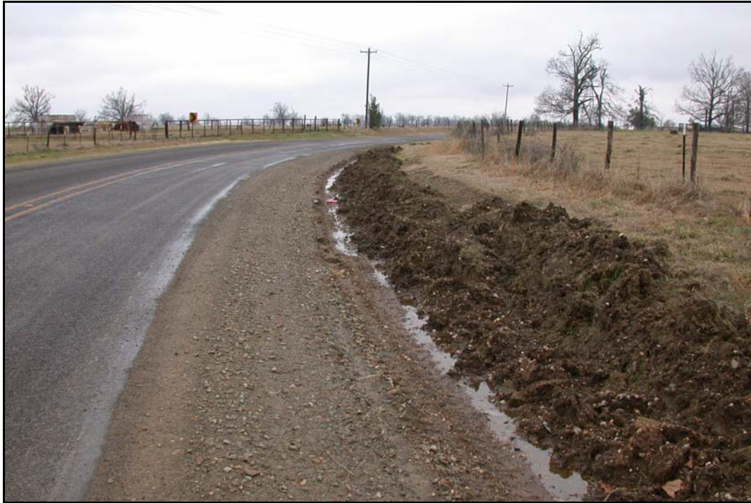
FIG. 5.26 Replenishing Repair at the Inside Horizontal Curve of an FM Road, Paris District (see Paris District Profile, Photo 23)
