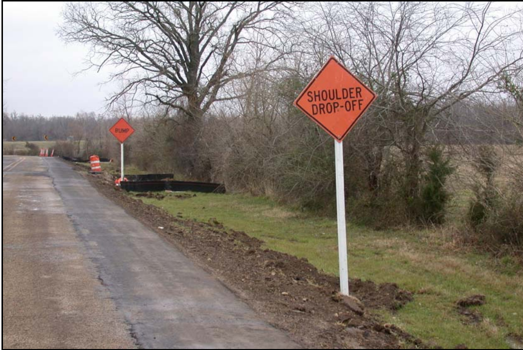
FIG 5.17 Shoulder Drop-off Sign, Construction Project, Paris District (see Paris District Profile, Photo 34)
