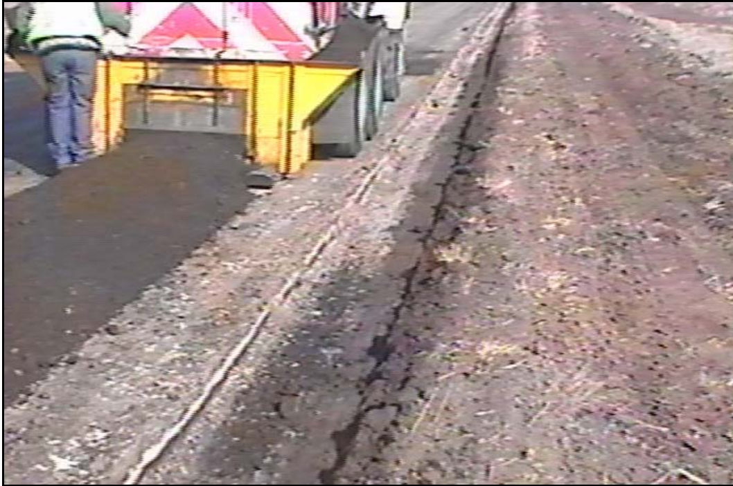
FIG. 7.9 Drag Box; Tow-Behind, Used for Delivering Windrow of Material to the Center of Pavement, Amarillo District
