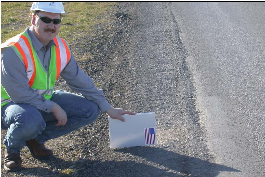
FIG. 7.35 Completed Edge Repair Project Using Midland Machinery Road Widener, Fort Worth District (see Fort Worth District Profile Photo 43)
