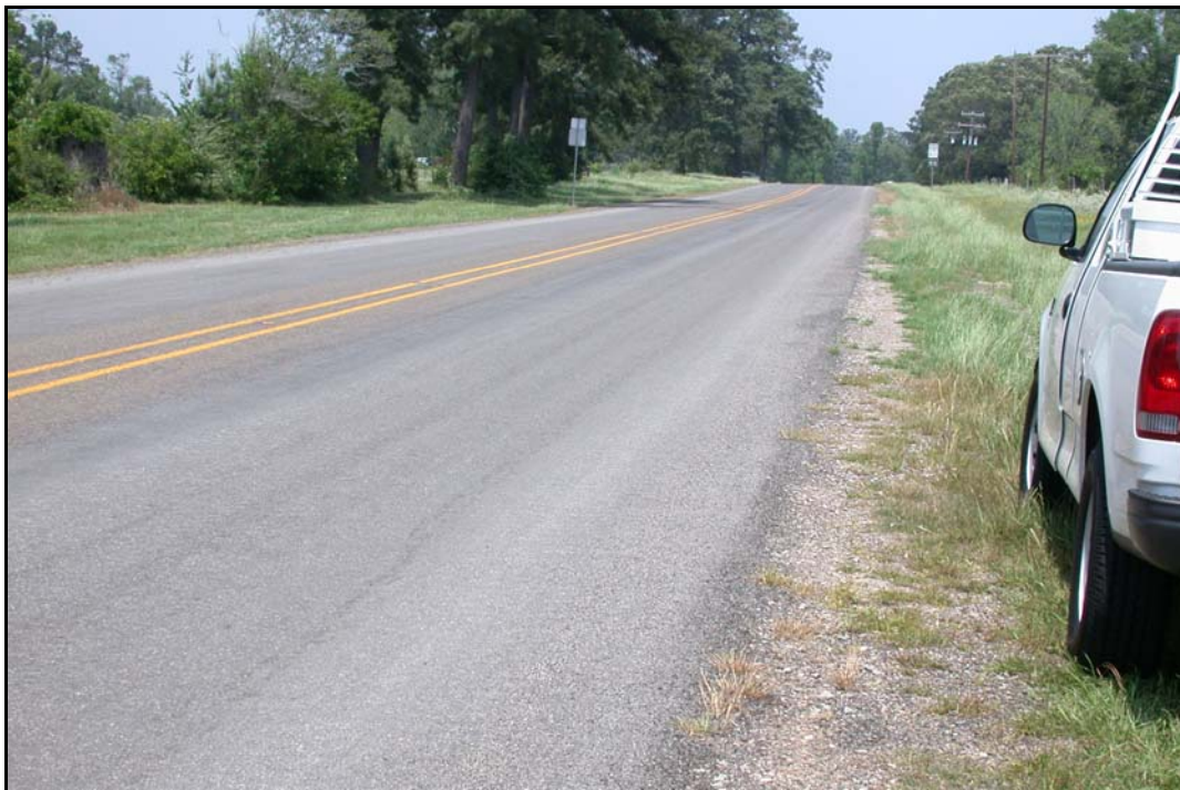
FIG. 6.16. FM 1005 Road Widening, Jasper County Texas, Beaumont District (see Beaumont District Profile, Photo 3)
