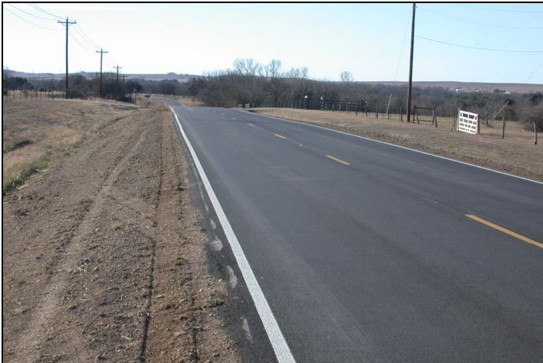
FIG 5.18 Typical Striping, Low-Volume FM Road, Fort Worth District (see Fort Worth District Profile, Photo 6)
