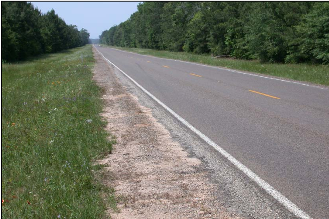
FIG 5.24 Cutting High Edges, Lufkin District (see Lufkin District Profile, Photo 14)
