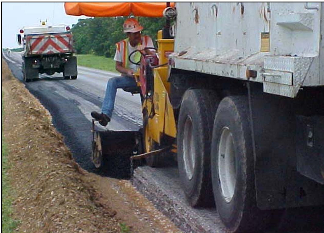
FIG. 7.32 LeeBoy 1200S Asphalt Maintainer for Edge Repair, Fort Worth District
