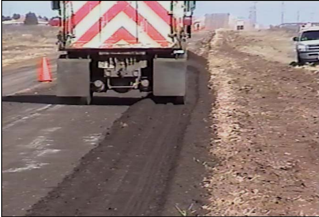
FIG. 5.28 District Forces Use Dump Truck Tires to Achieve Ordinary Compaction for Edge Repair, Amarillo District
