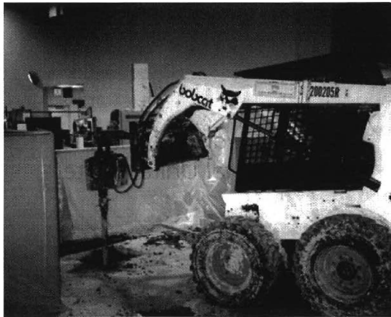
Figure 5.3 5-foot 6-inch-wide, 6-foot 9-inch-high Specialty Rig Drills Holes up to 60-inch Diameter and 75-foot Depth (Source: S & W Foundation, Richardson, Texas)
