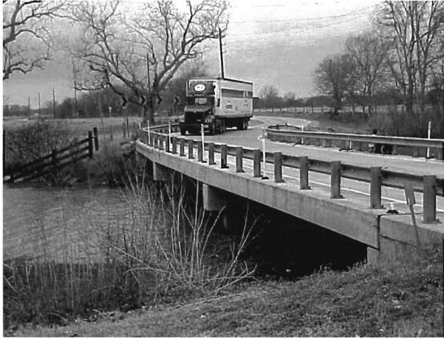
Figure 5.14 Off-system Bridge on Hunt Road at Bessie's Creek
