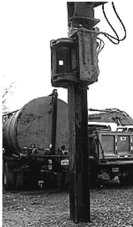
Figure 5.5 Robotic Vibratory Pile Driver Attached to an Excavator
