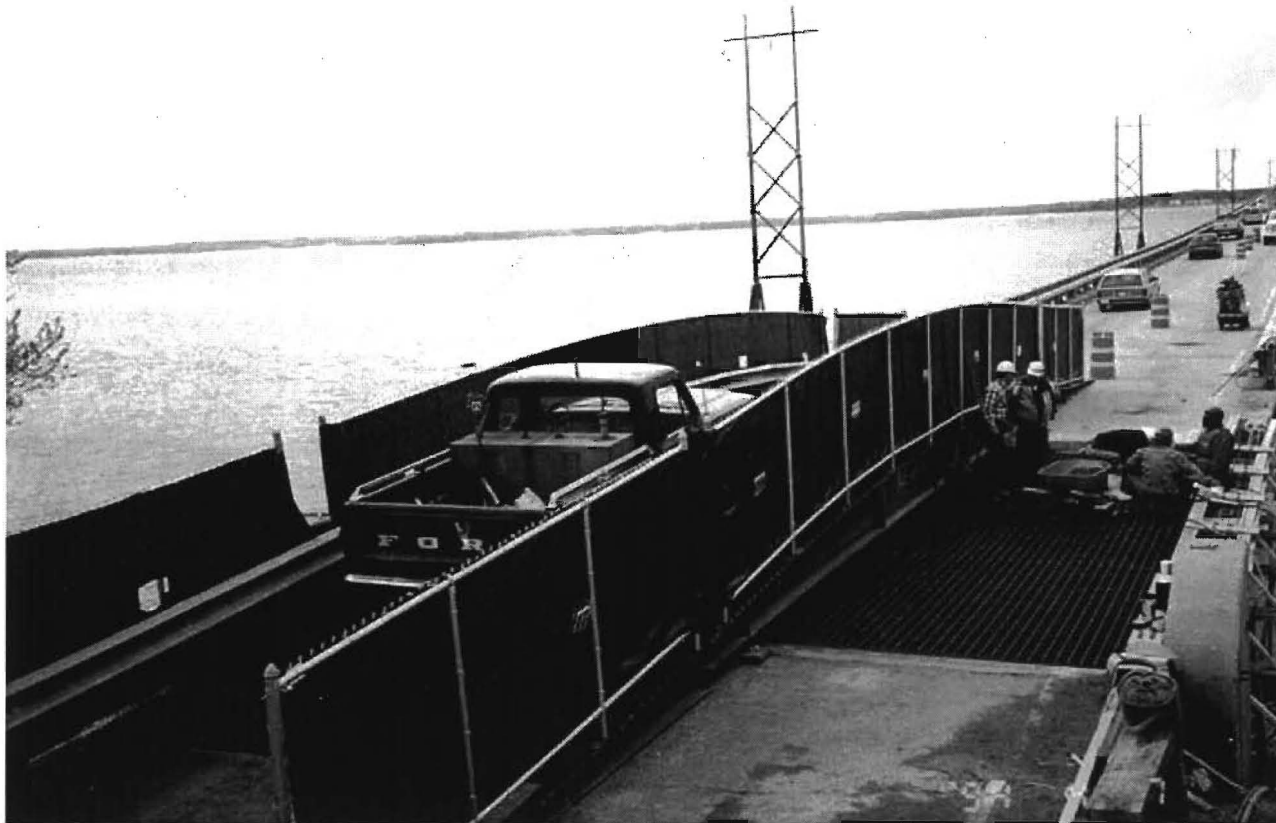
Figure 5.11 Temporary Bridge in Use During Bridge Reconstruction
