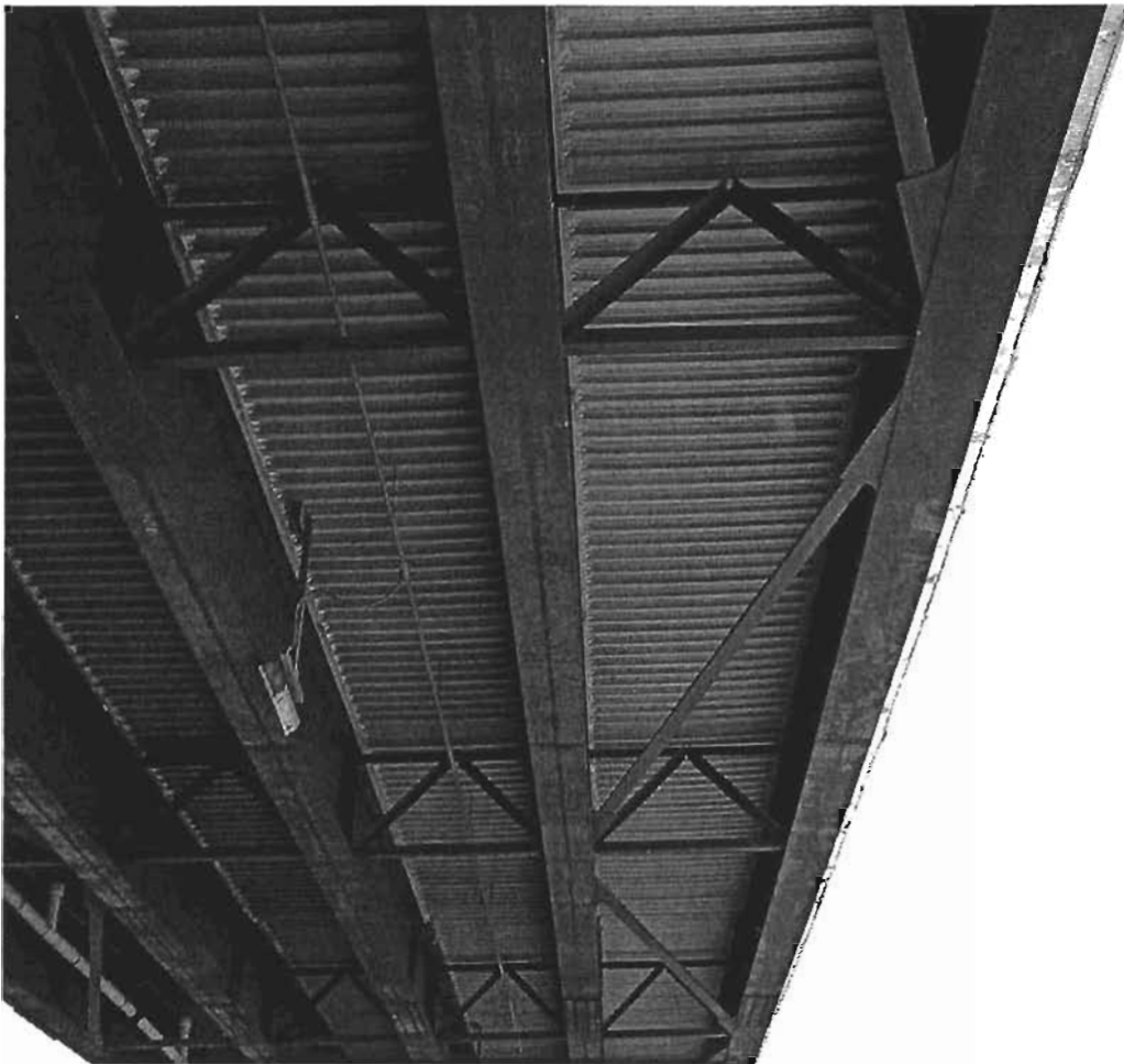
Figure 1.1 Metal Deck Forms viewed from the underside of a Bridge
