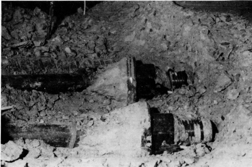
Fig. 6.17 Individual cones of crushed concrete in front of the anchorage devices--bolt spacing = 5 in.
