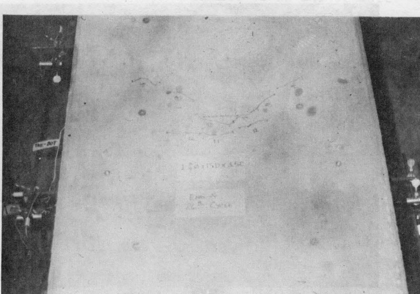
(b) Cracking at end of first set of loading cycles
