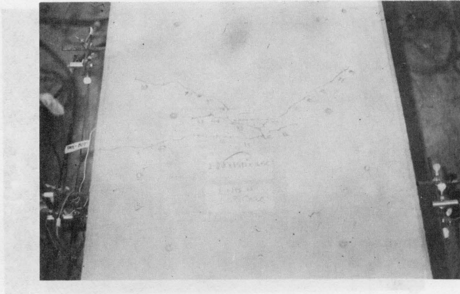
(c) Cracking at end of second set of loading cycles
