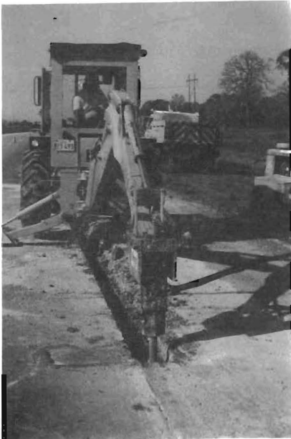
Fig 4.2. Breaking the CTB with an air hammer.
