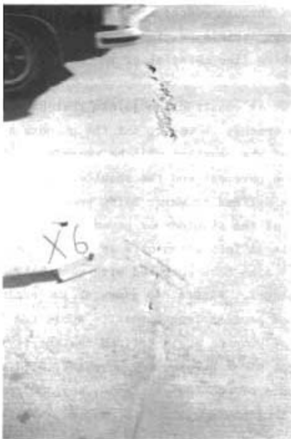
Fig B.6. Severe spalling.
