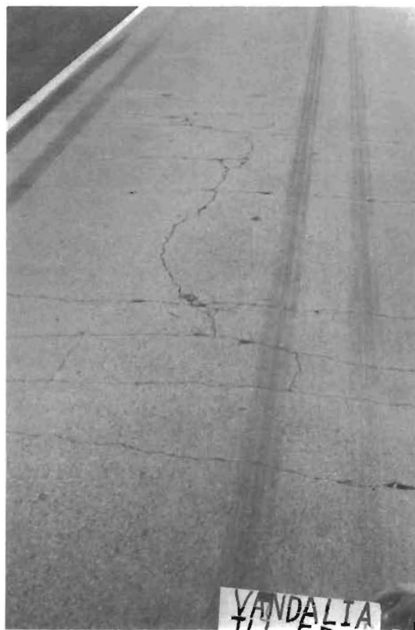
Fig B.10. Minor punch out.
