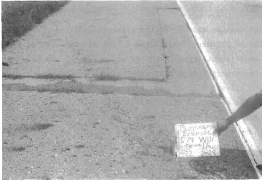
Fig B.16. Subsurface drain installed.
