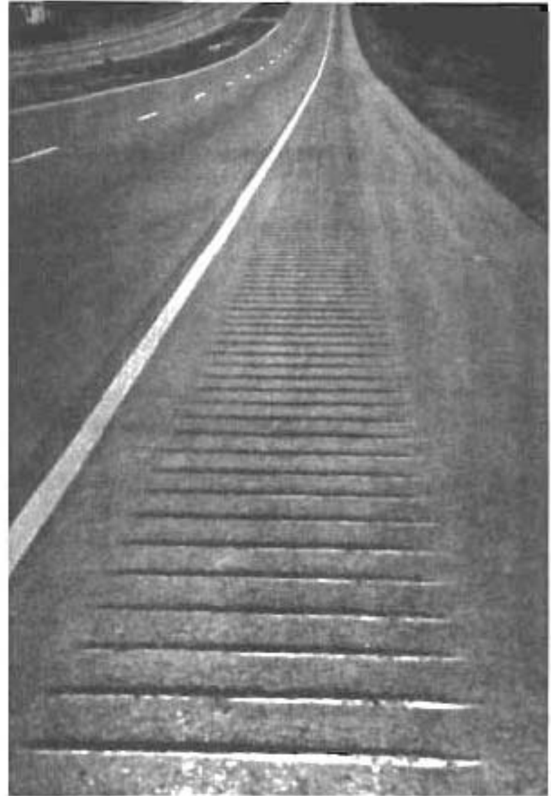
Fig. 2.4 Grooves 36 in. (900 mm) in length pressed into hot HMA
