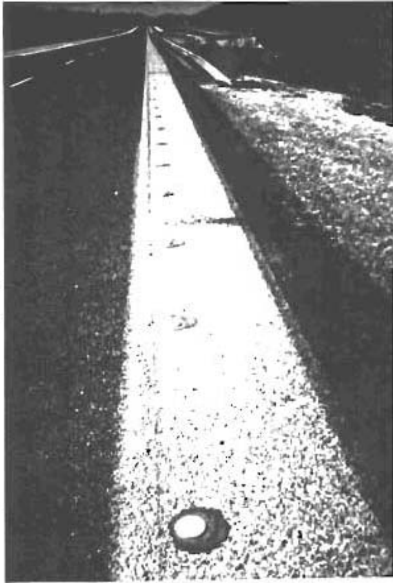
Fig. 2.3 Traffic buttons installed 5 ft (1.5 m) center parallel to the outside lane edge line
