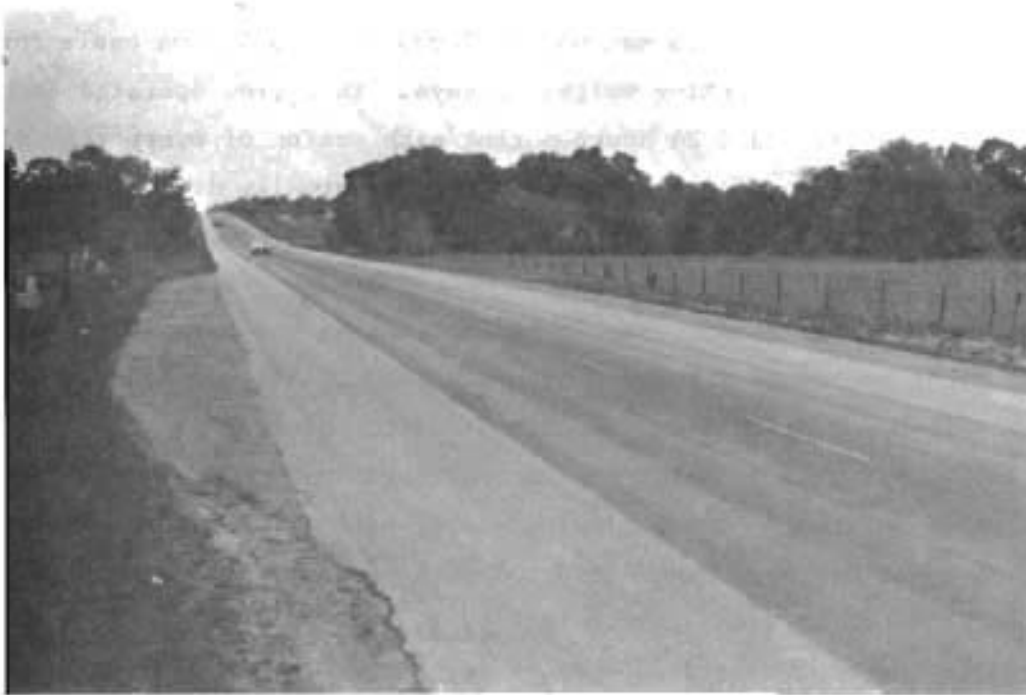
Fig 2.2a. Site preparation for typical static weight survey station.
