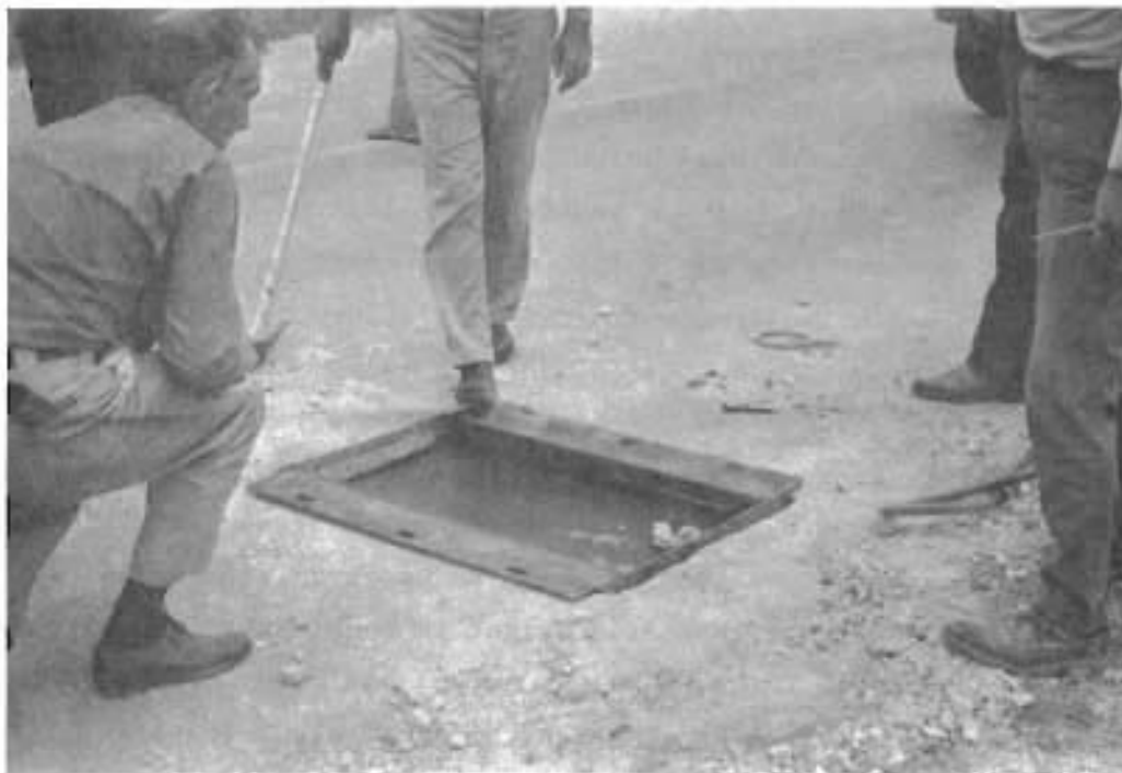
Fig 2.2b. Metal-lined pit for loadometer application.
